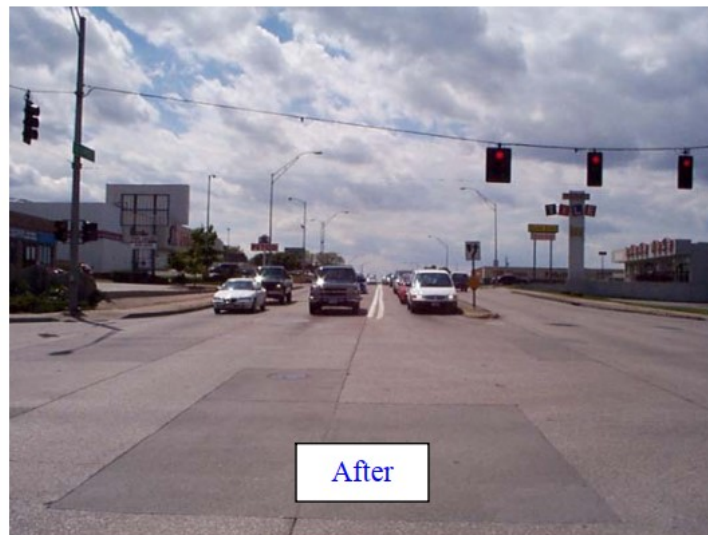
Figure 2.1 Left-turn lane line treatment at 48th and 'O' St, line width increased from 0.3 feet to 1.5 feet. [Khattak et al., 2004]
