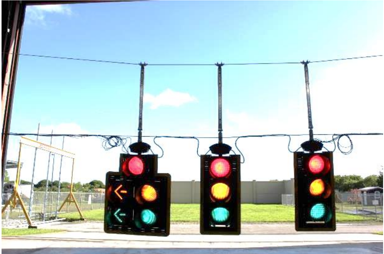
Figure 13: Signal assemblies installed on test frame (before testing)
