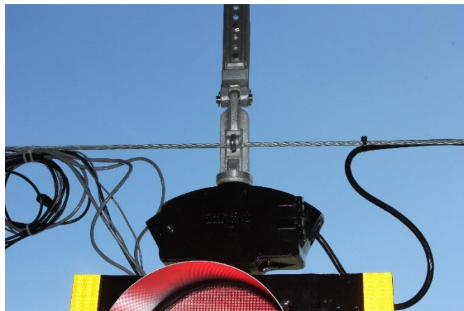
Figure 15: Close-up view of the pivotal hanger connection
