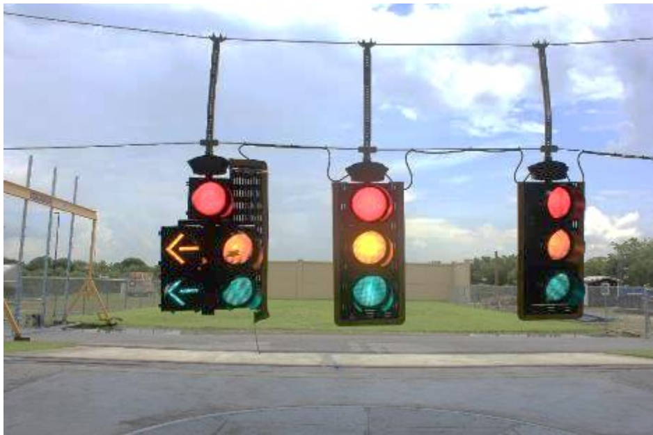
Figure 41: Traffic signals after completion of 130 mph test
