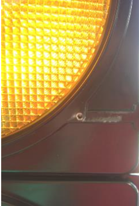
Figure 89: East 3-section signal with sheared off visor screw
