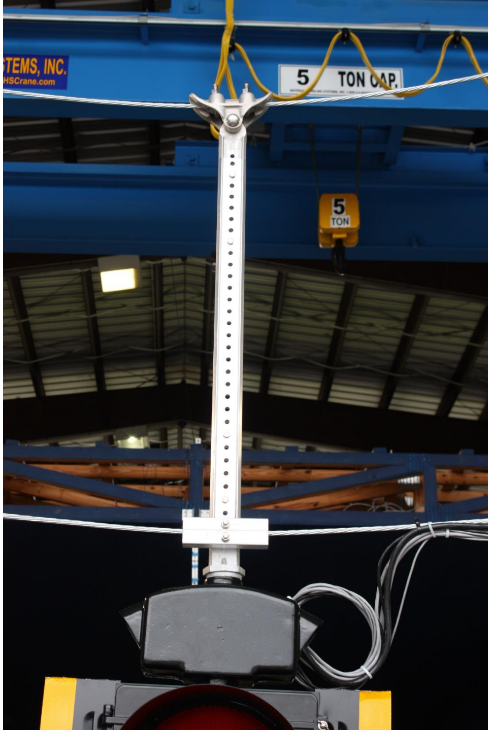
Figure 164: Hanger connection after test
