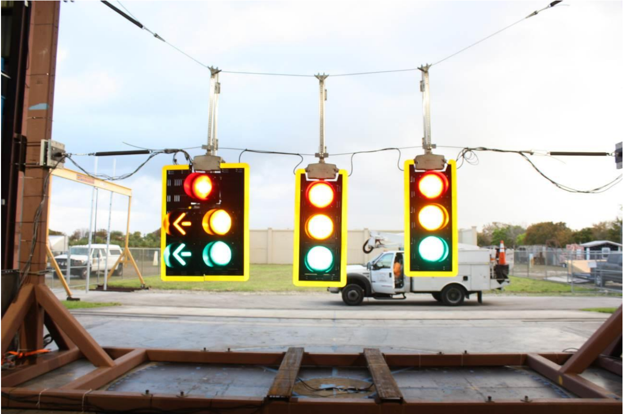
Figure 135: Signal assemblies installed on test rig (before testing)
