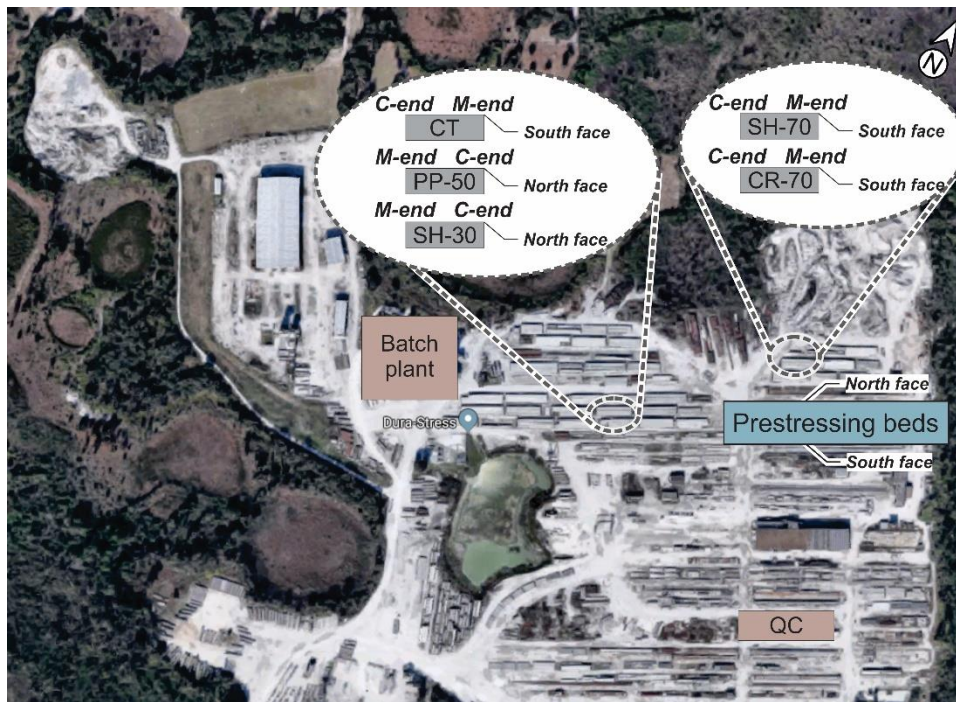
Figure 4-17 Girder location within the precast plant
