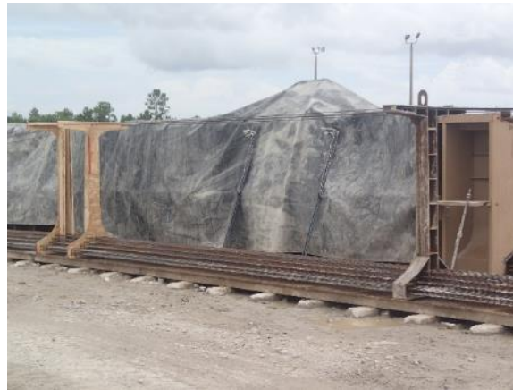
Figure 4-8 Prestressing strands after tension was applied
