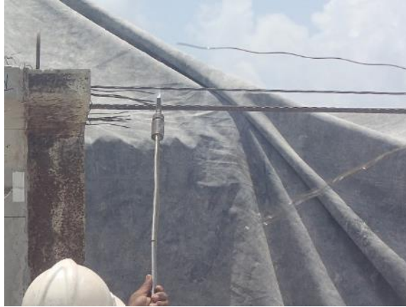
Figure 4-15 Flame cutting of prestressing strands
