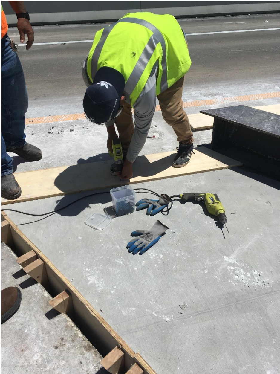
Figure 2-17: Plywood being fastened on UHPC joint to curb water loss
