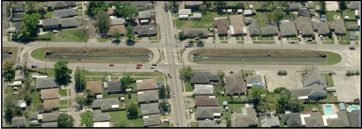
Figure 2-11: MUT intersection with water retention ponds in median in New Orleans, Louisiana (Reid et al., 2014)
