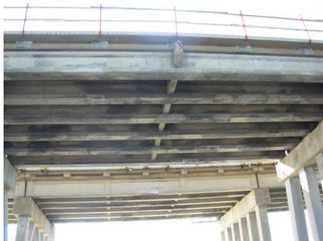
Figure 1. Typical Deterioration on the Lesner Bridge
