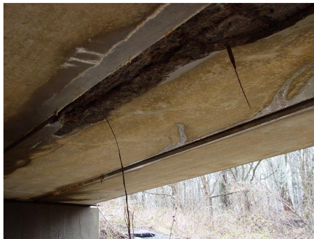
Figure 2. Typical Corrosion Damage on Aden Road Bridge
