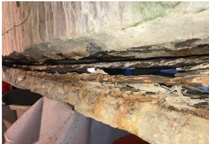
Figure 70. Strand Condition for Box Beam 4 West Side
