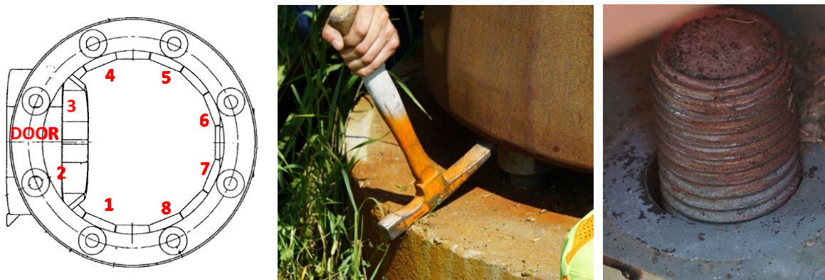
Figure 3.3.16 Rod numbering (left), checking washers for looseness (center), and prior copper anti seize lubrication on rod (right)
