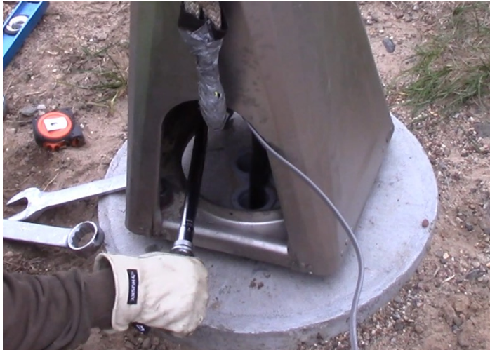
Figure 3.3.5 Applying verification torque
