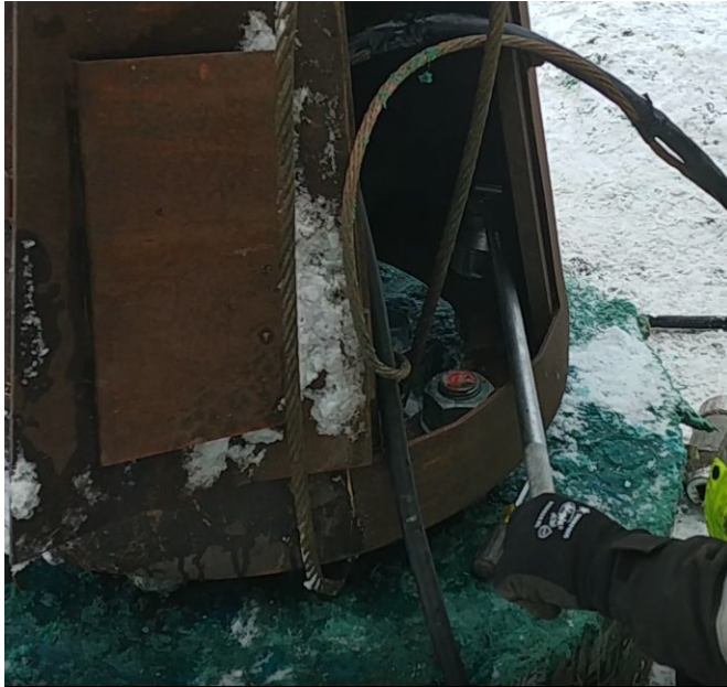
Figure 3.3.10 Manual wrench installation tightening of HMLT anchor rods
