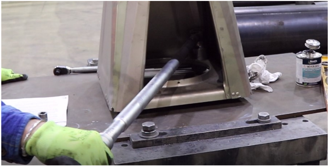
Figure 3.3.8 Final verification torque on the structure installation
