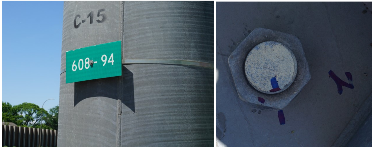
Figure 3.2.14 I-94-608 Post (left) and 1/12 turn on nut #8 (#2 in star pattern) (right)
