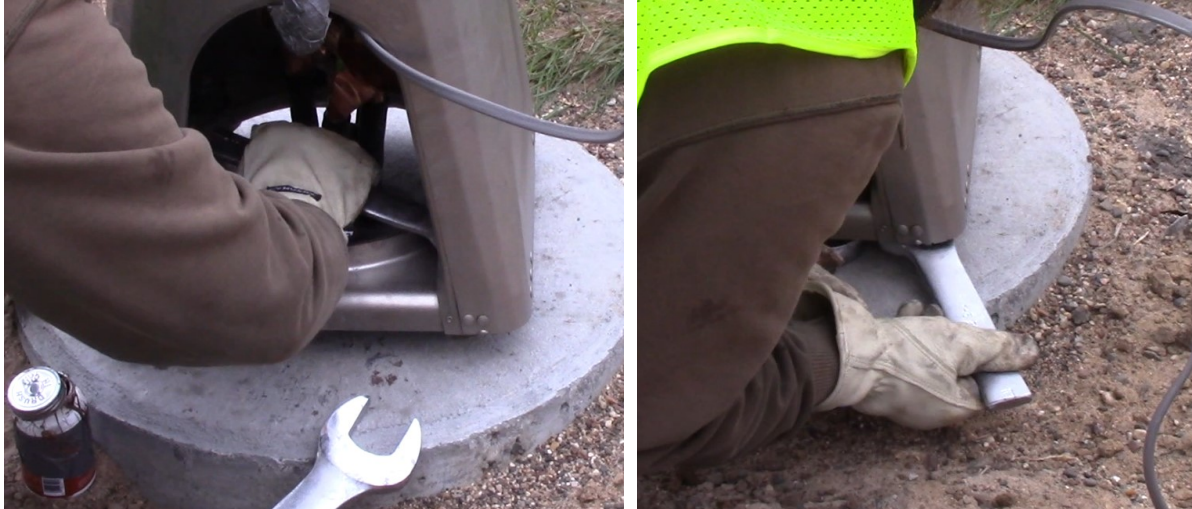
Figure 3.3.3 Snugging top nuts (left) and snugging leveling nuts (right)
