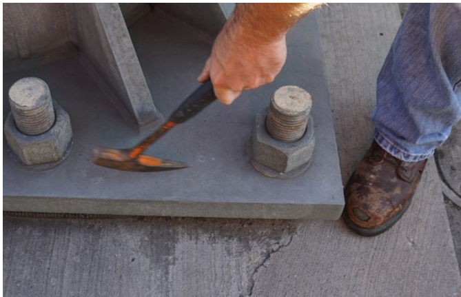
Figure 3.1.1 Checking for clamping force in connection
