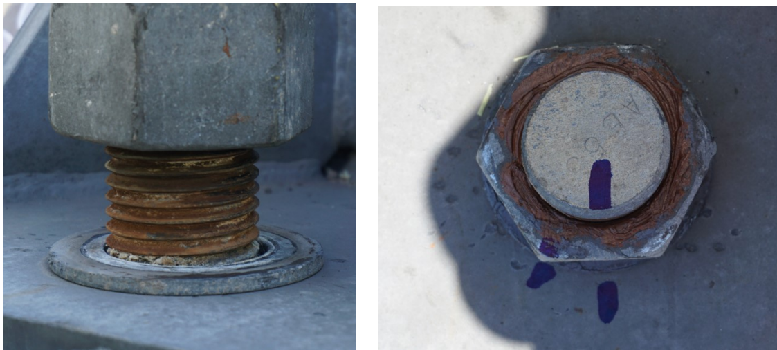
Figure 3.2.13 General condition of anchor rods (left) and sample turn-of-nut verification (right)
