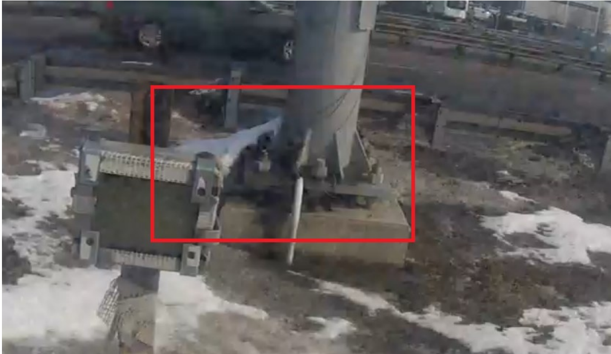
Figure 4.2.5 Snow and ice piled on anchor rod gauges
