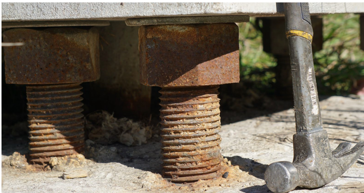
Figure 3.2.9 Large standoff distance on I-494-153 structure
