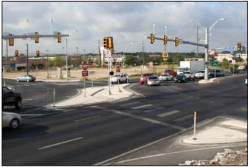
Signalized RCUT intersection in operation near San Antonio, TX showing a pedestrian "Z" crossing.
