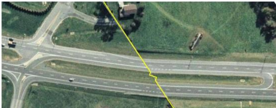
Merge-controlled RCUT intersection on US-15 in Emmitsburg, MD.
