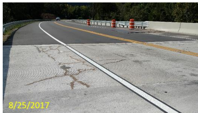
Figure 6 – Typical cracks in the acute corner of Span 1.
