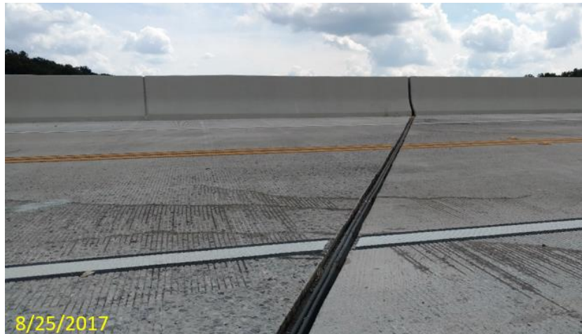
Figure 41 – Old photo showing cracks thru expansion joint between Spans 1 and 2.
