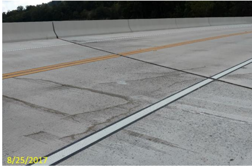
Figure 39 – Old photo showing cracks in eastbound lane at Span 2 end.
