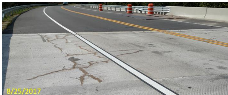
Figure 15 – Additional cracks along SR299 bridge (westbound lane shoulder of Span 1).
