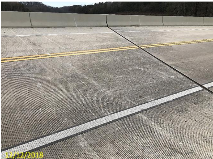
Figure 40 – New photo showing cracks in eastbound lane at Span 2 end.
