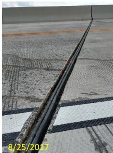
Figure 7 – Typical longitudinal cracks at the expansion joint.
