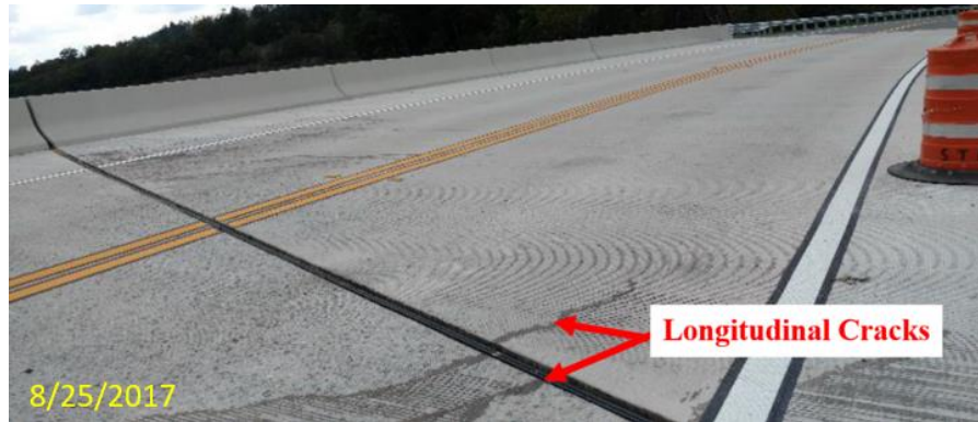
Figure 13 – Longitudinal cracks at the expansion joint on SR299 bridge (eastbound lane of Spans 1 and 2).
