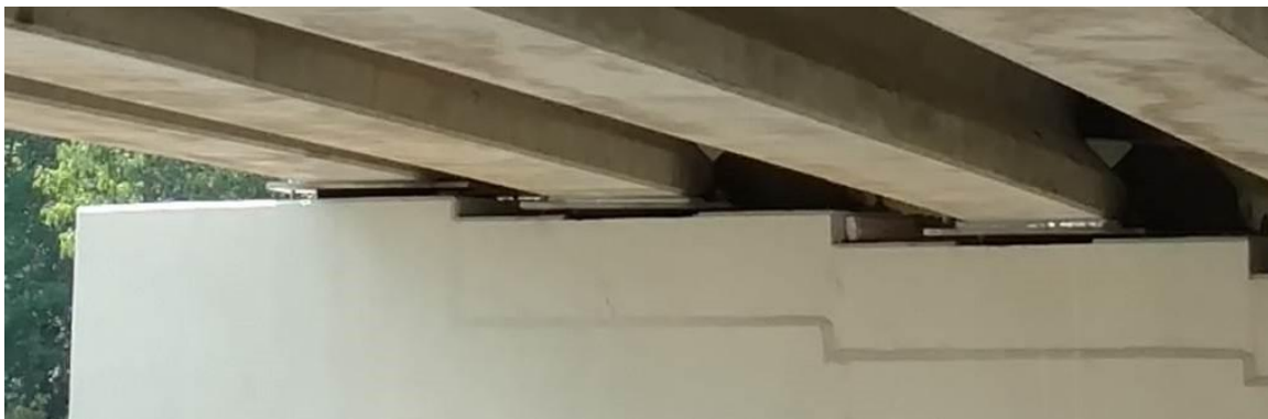
(d) Bearing conditions enlarged from the photo shown in (c).
