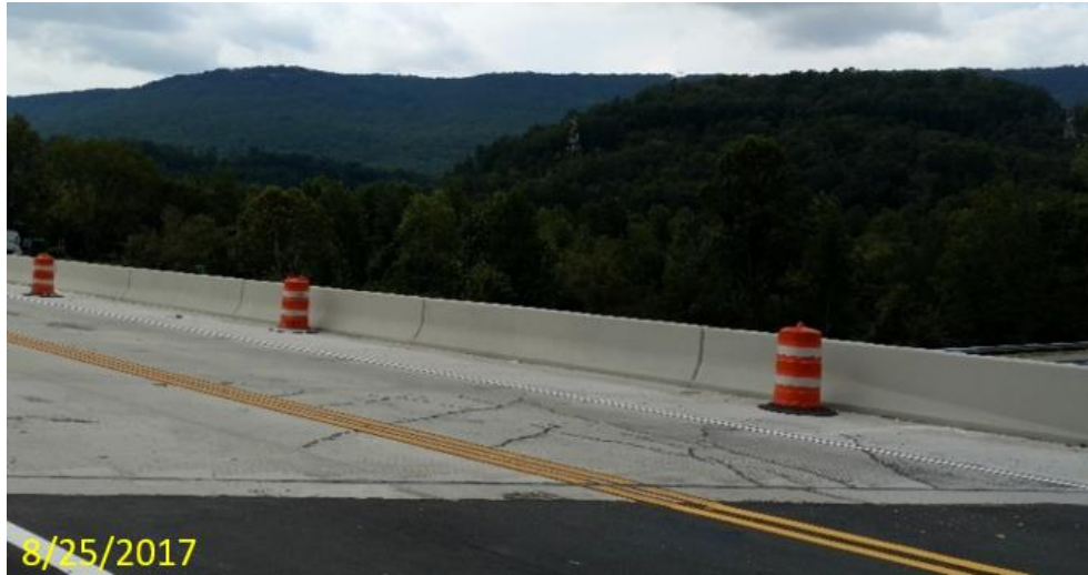
Figure 37 – Old photo showing cracks at eastbound corner of Span 2.
