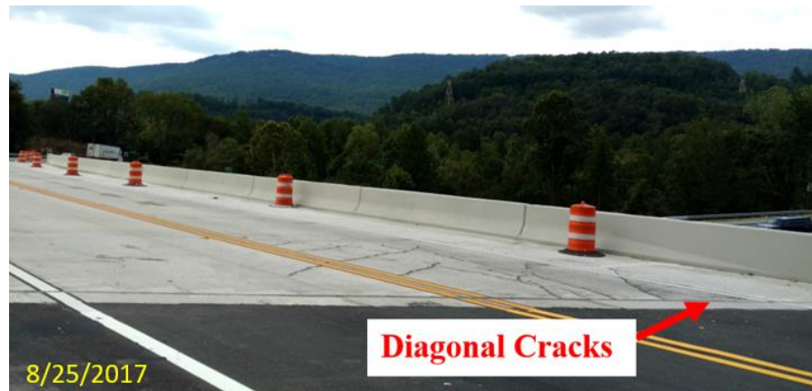
Figure 14 – Typical diagonal corner cracks on SR299 bridge (eastbound lane of Span 2).
