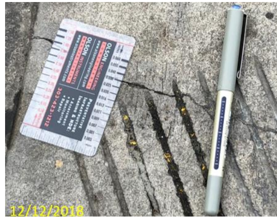
Figure 35 – Crack width measurement (0.030 in. or 0.76 mm).
