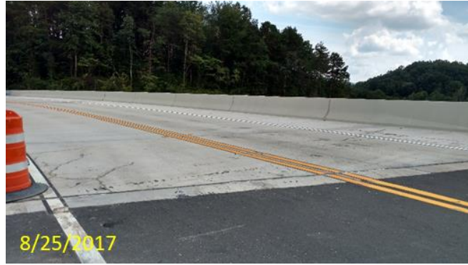
Figure 5 – Typical deck corner cracks in Span 1.
