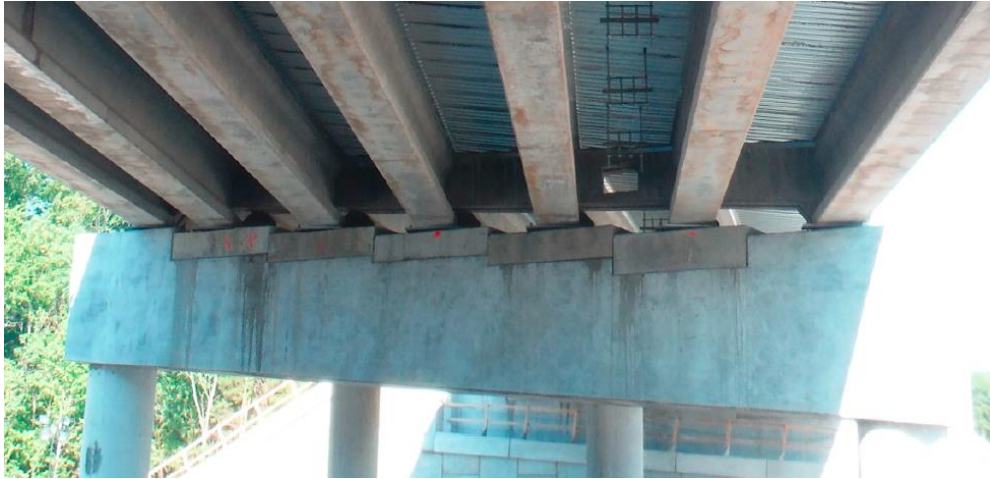
(b) Bearing conditions during the first bridge inspection by GDOT (GDOT BIR, 2017).
