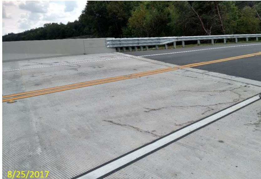
Figure 43 – Old photo showing cracks at the obtuse corner of eastbound Span 1.
