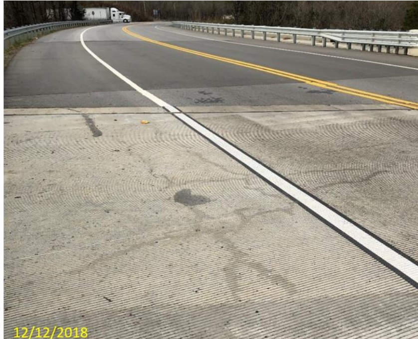
Figure 46 – New photo showing cracks at the acute corner of westbound Span 1.
