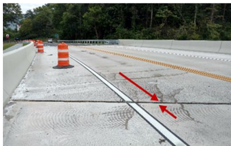
Figure B-4: Expansion joint at Intermediate Bent 2.
