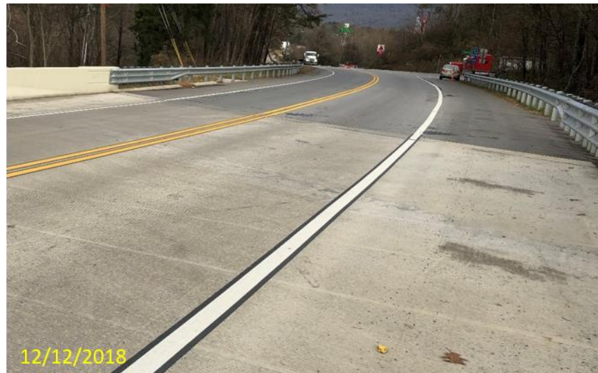
Figure 48 – New photo showing cracks from westbound lane of Span 2.
