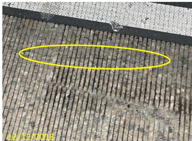
Figure 31 – Untreated longitudinal cracks without epoxy coatings.
