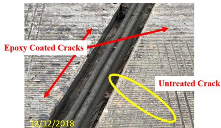
Figure 29 – Crack through the expansion joint.
