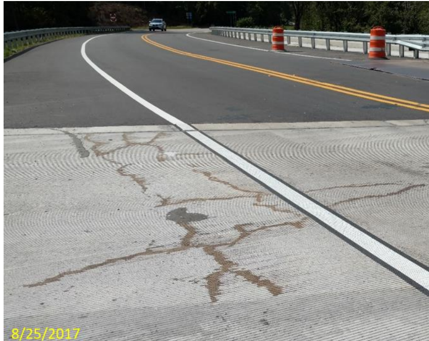
Figure 45 – Old photo showing cracks at the acute corner of westbound Span 1.
