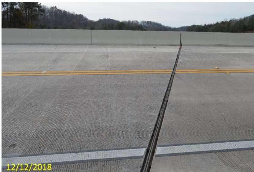
Figure 42 – New photo showing cracks thru expansion joint between Spans 1 and 2.
