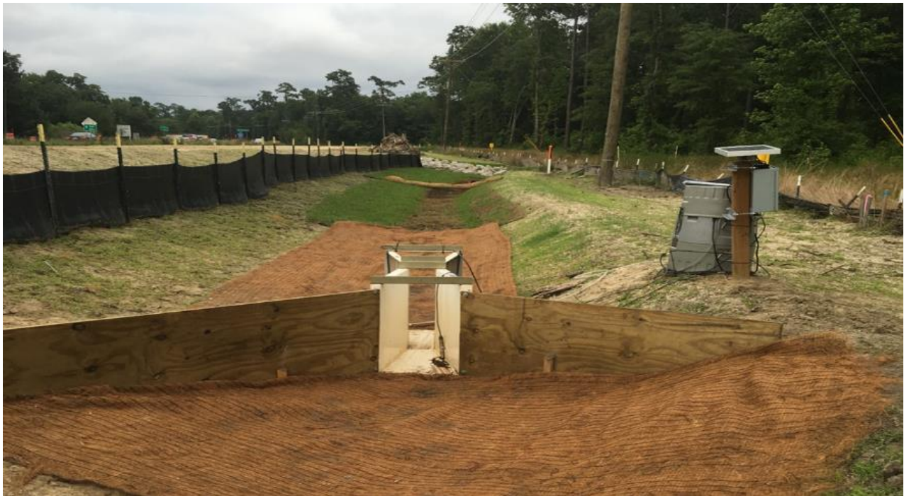
Figure B.6. Coastal research station showing instrumentation and Parshall flume.
