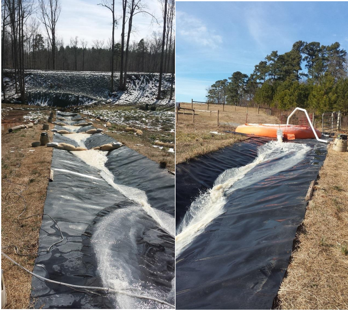
Figure A.1. Channel Design. On left, upstream view of channel from bottom. On right, downstream view of channel from tank outlet during experimentation.
