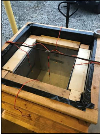
(a) assembling the formwork
