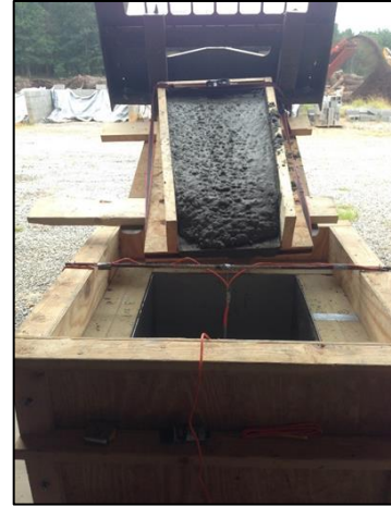
(c) concrete placement
