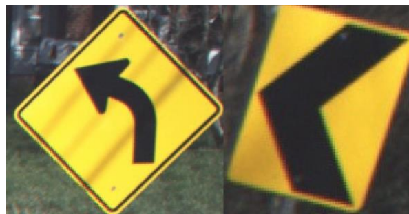
FIGURE 3-3. Photo. Examples of curve signs with diamond and rectangular shapes
