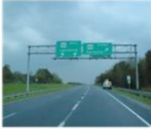
A. Subfigure of sign-bridge-mounted
