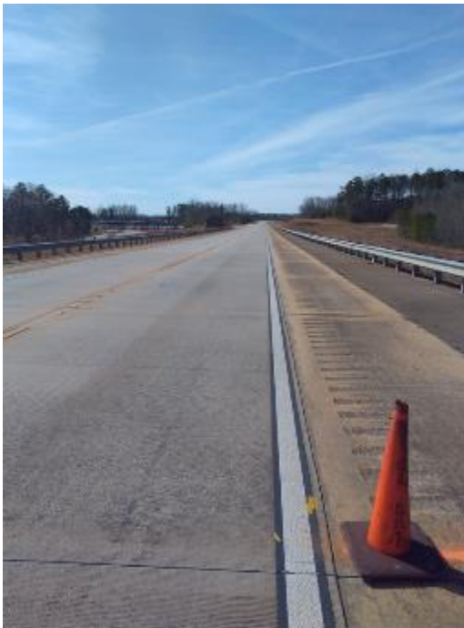
A. Subfigure of concrete test section
