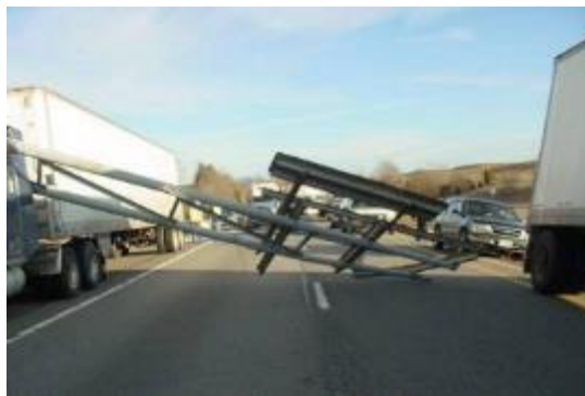
Figure 3-3. Photo. Example of overhead sign failure (FHWA, 2013).
