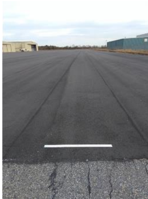
B. Subfigure of asphalt test section
