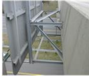
C. Subfigure of bridge-mounted
