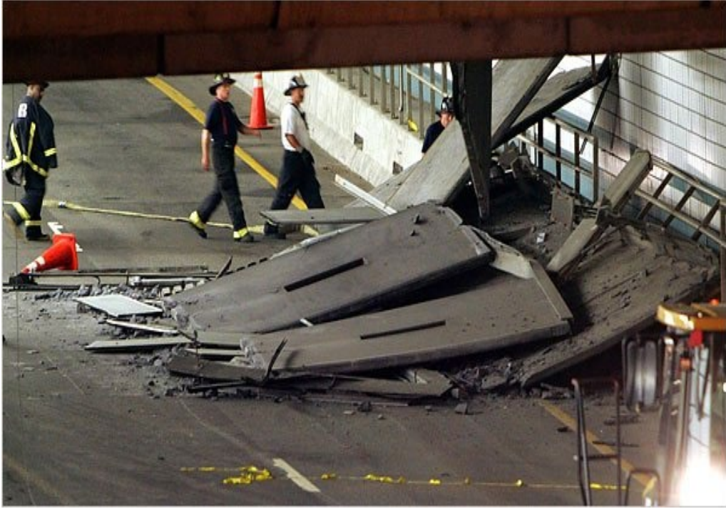
Figure 2. Photo. Aftermath of Big Dig Collapse (Cornado Common Sense, 2008)
