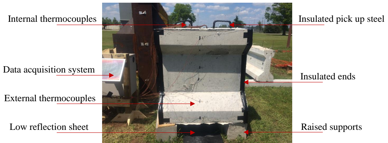
Figure 3.7 - Fully instrumented Type IV girder segment – Norman, OK
