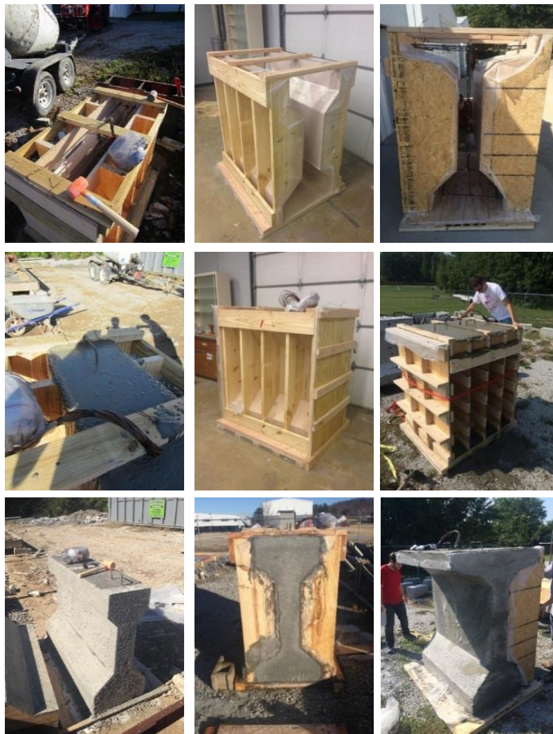
Figure 3.1 – Girder segment construction process
