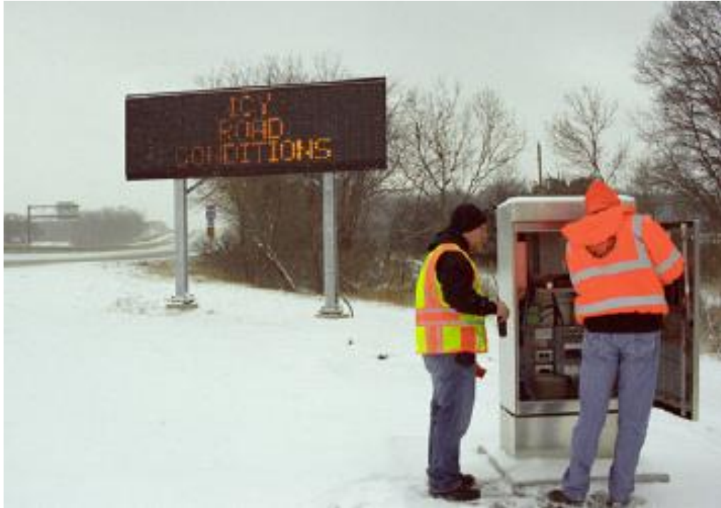
Figure 2-18 Fixed traveler message sign warning drivers of icy road conditions in Kansas (KDOT, 2017)
