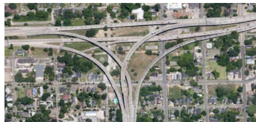
Interchange of Interstates 10 and 110 in downtown Baton Rouge.
