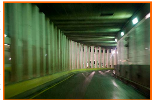
Entrance photograph of the Detroit—Windsor International Tunnel
