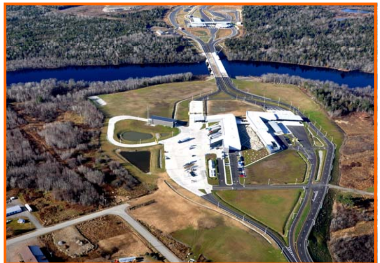
The above photograph is an aerial shot taken of the new Calais—St. Stephen Border Port of Entry
