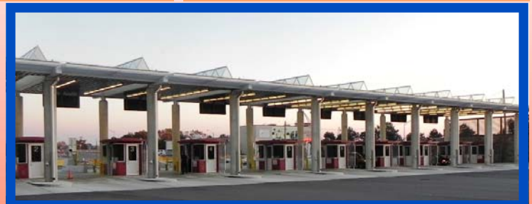
The Queenston Port of Entry was the second stop on the bus tour. Shown above was the passenger vehicle processing pill boxes that were recently constructed.
