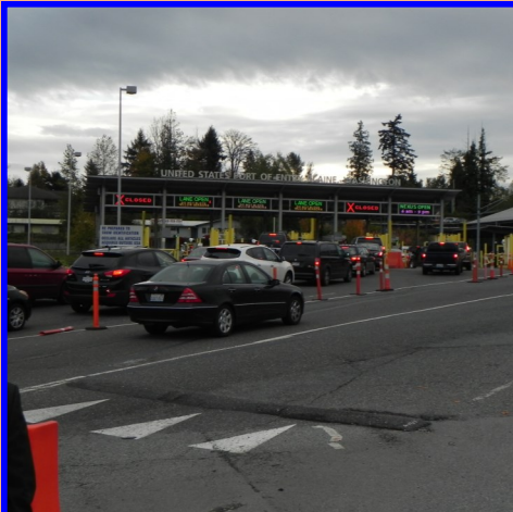
A motorist's view as they approach the U.S. Inspection Booths of the Pacific Highway facility.
