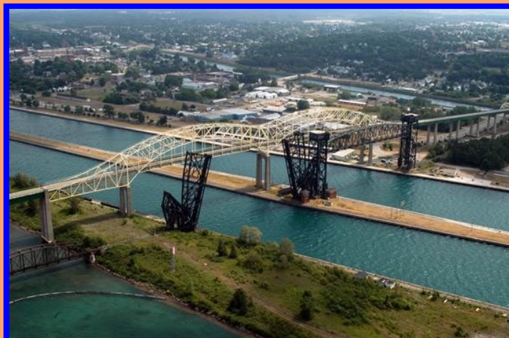
An aerial view of the Sault Ste. Marie bridge that GSA toured as part of their Michigan Port of Entry Tour.
