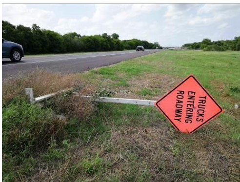
(a) Wood Traffic Sign Fallen Down
