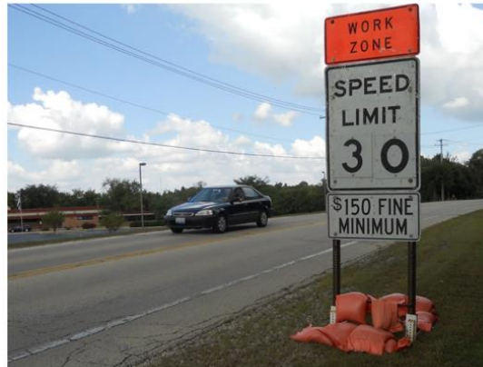
Figure 14. Sandbags on skid as ballast to resist high speed wind forces
