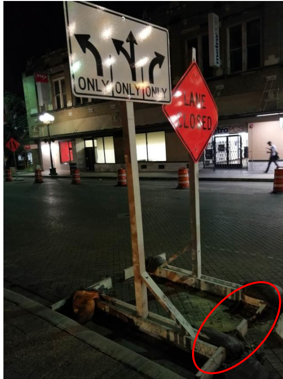
Rot Damage of a wood traffic sign in San Antonio, TX Figure 51. Performance Check of Traffic Signs in San Antonio, TX
