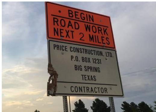
(b) Traffic Sign Partial Damage
