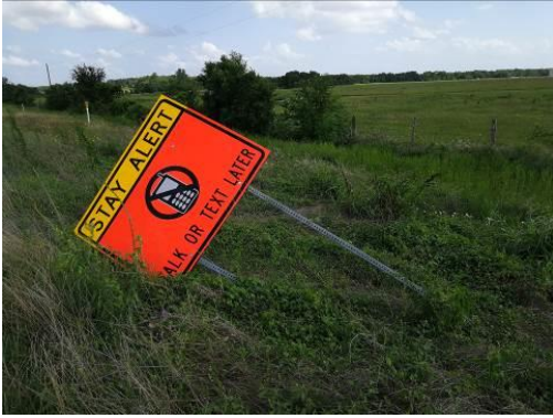
(a) Traffic Sign 2000 Fallen Down
