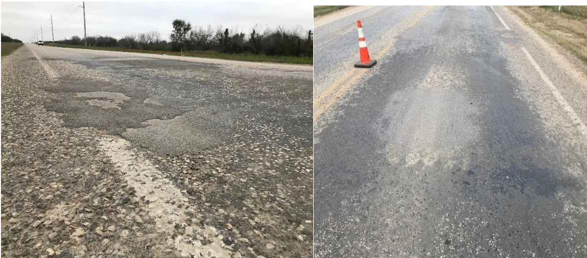
Figure A.3. Patches in FM 468 - La Salle County
