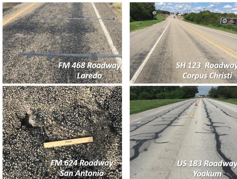
Figure 6.1. Distresses in Roadways of Eagle Ford Shale Region.
