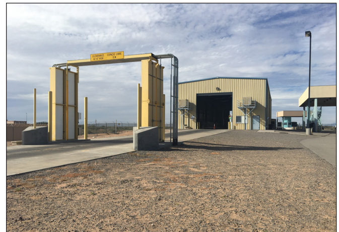
A freight x-ray scanner at the Santa-Teresa crossing in New Mexico. Source: J. Davis
