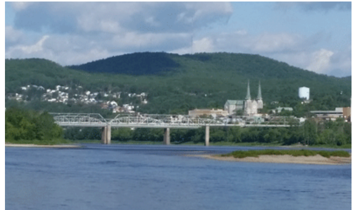
The Madawaska-Edmundston Bridge. Photo credit: fixitnowmaine.org
