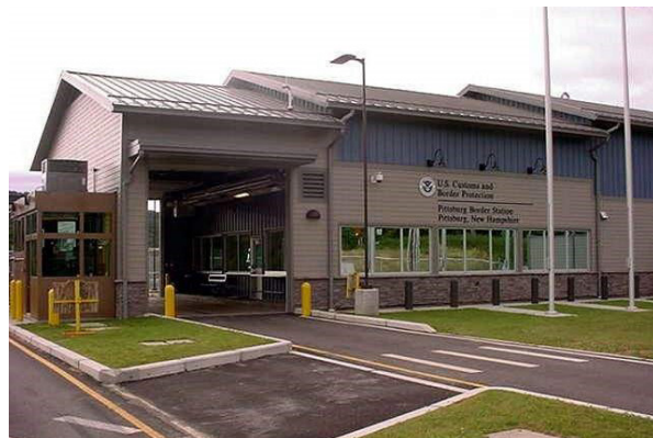
U.S. Customs Border Protection facility at Pittsburg, NH.
