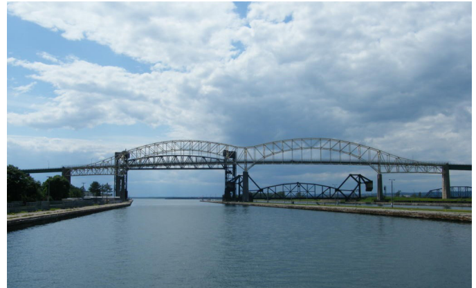
Sault Ste. Marie International Bridge. Source: www.wnmufm.org
