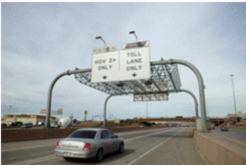
(Picture showing the left lane is for free HOV 2+ and the right lane is for tolled traffic.)
