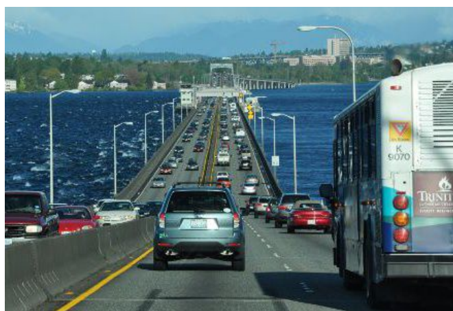
Figure 2. SR 520 Bridge (Source: Washington State DOT)
