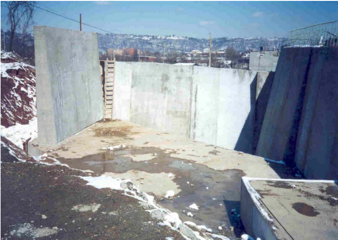
Figure 10-18. CIP abutment with integral wingwalls
