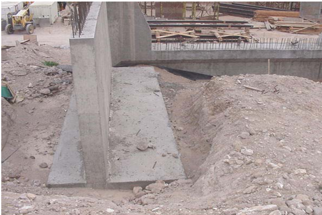
Figure 8-5. Abutment/wingwall footing, I-10, Arizona.
