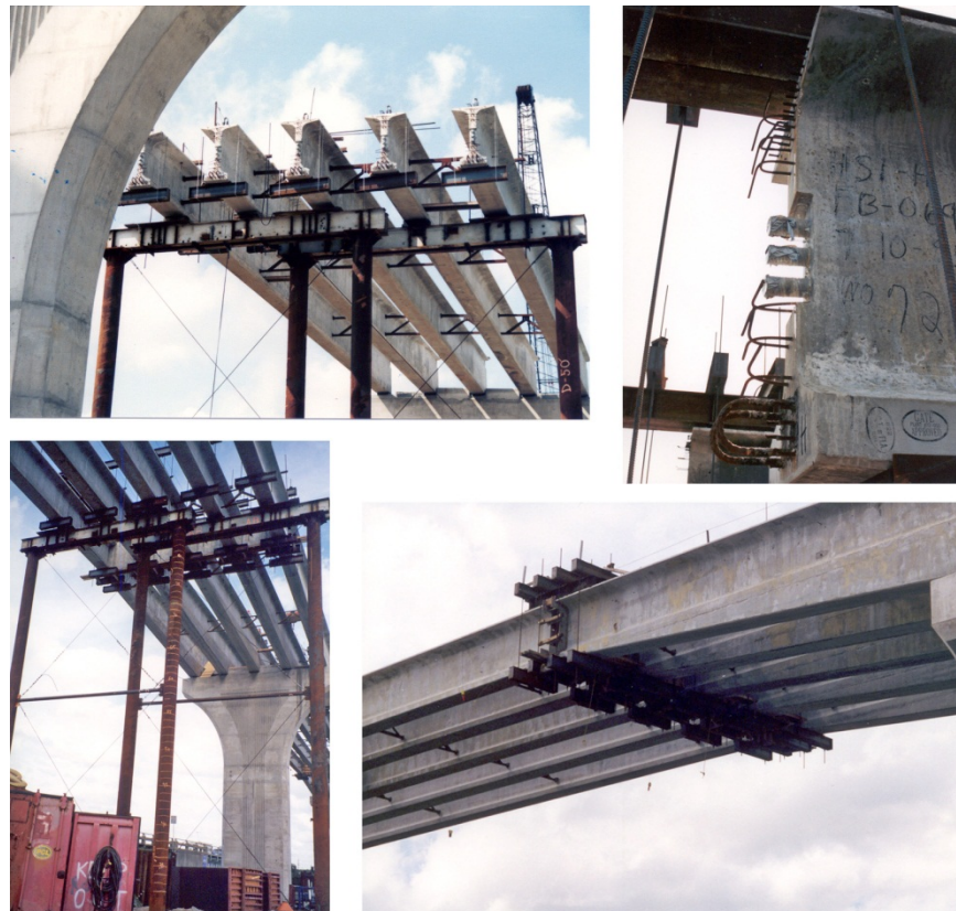
Figure 1.7 - Spliced Haunched I-Girder of Main Span Unit
