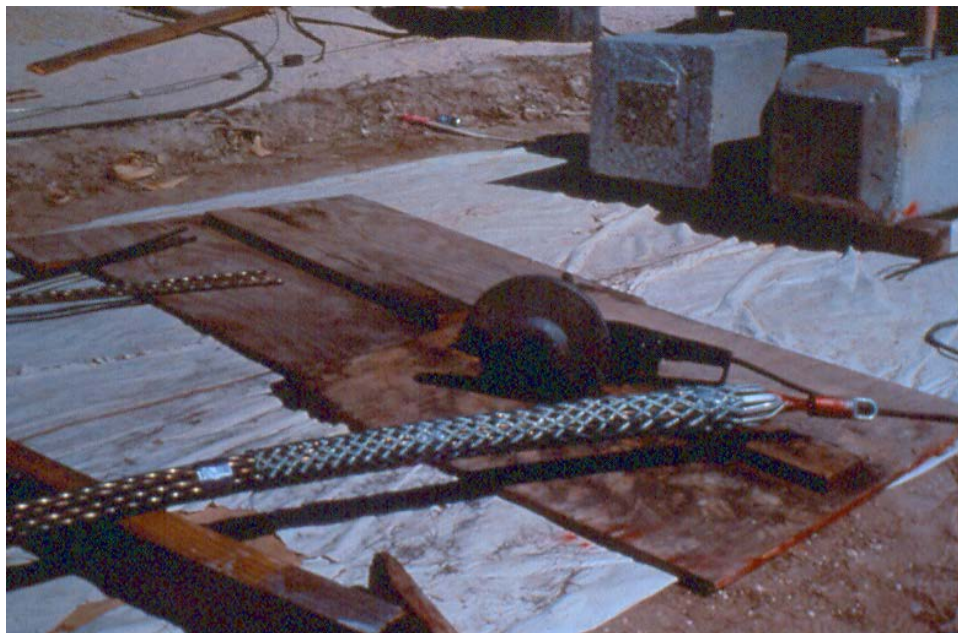
Figure 3.26 - Steel wire sock for installing multi-strand tendon
