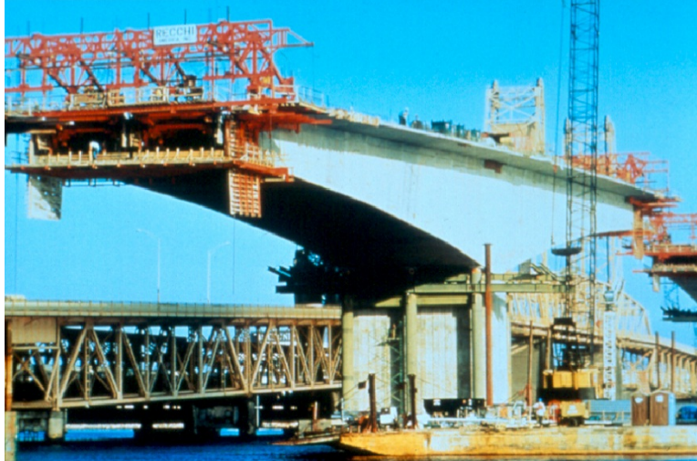
Figure 1.17 - Cast-In-Place Segmental Construction using Form Travelers
