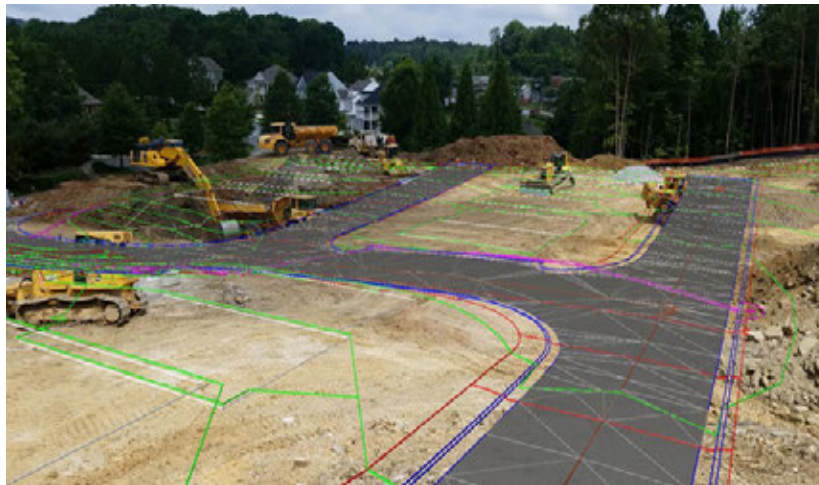
Highway designers and builders can view design data overlaid on a real-world, existing construction site. Here, the overlaid lines show the wireframe and surface geometry from the design data.
