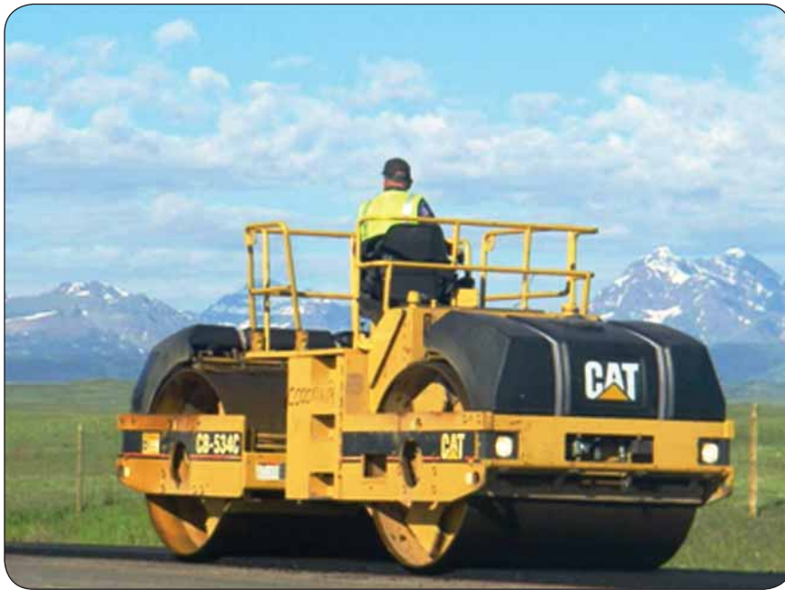
Blackfeet Tribe paving project — Tribal personnel operating breakdown roller from the Rocky Mountain Region's equipment pool
