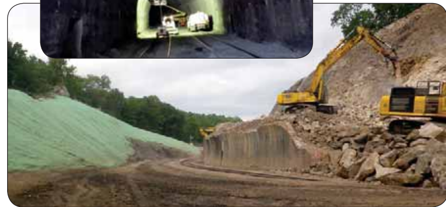
Example of an open cut tunnel, full excavation of rock and soil from the top of the tunnel, fully exposing the track, creating a valley. A portion of the original brick lining of the tunnel wall is visible on the right — Shoofly Tunnel near Markelton, Pennsylvania
