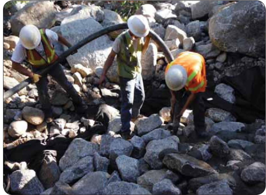
Grout installation — Kings Canyon National Park, California
