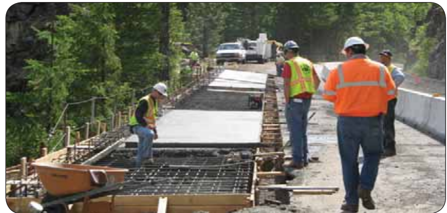
FLH Staff Project Reviews, North Umpqua Highway, Umpqua National Forest, Oregon
