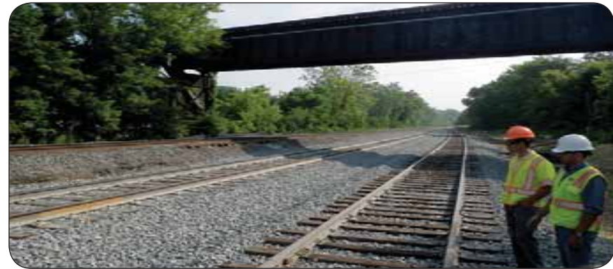
View of lowered tracks, original track height to be removed is visible on the far left — track under the W&LE Railroad Bridge, Kent, OH
