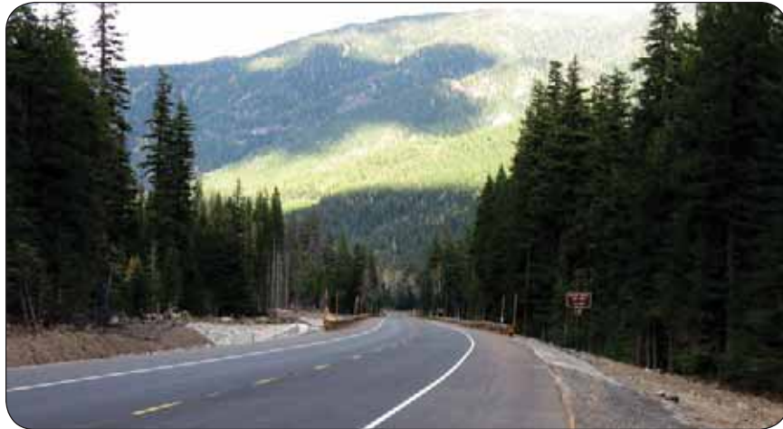
Raised roadway, Highway 35, Oregon (see Other Title 23 Project Summary pg 21)
