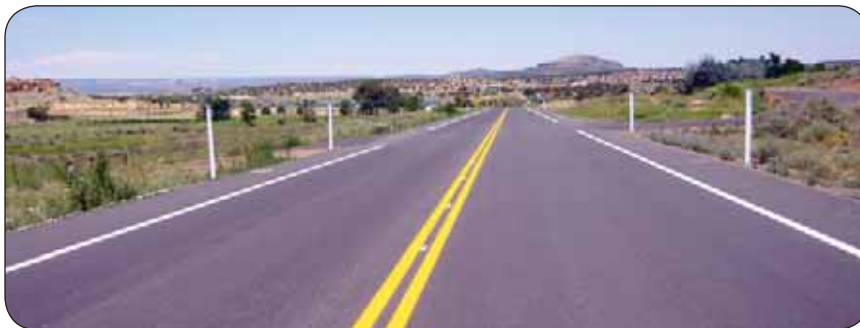
Project included improvements to pavement markings, approach roads, signs, and delineators
