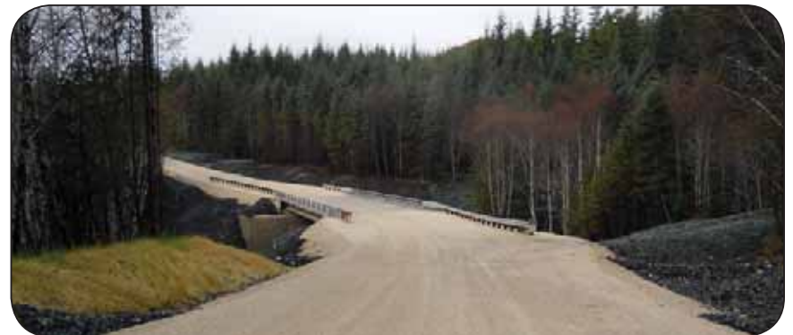
View of approach, Jenny Creek Bridge, Alaska (see FH Project Summary pg 18)
