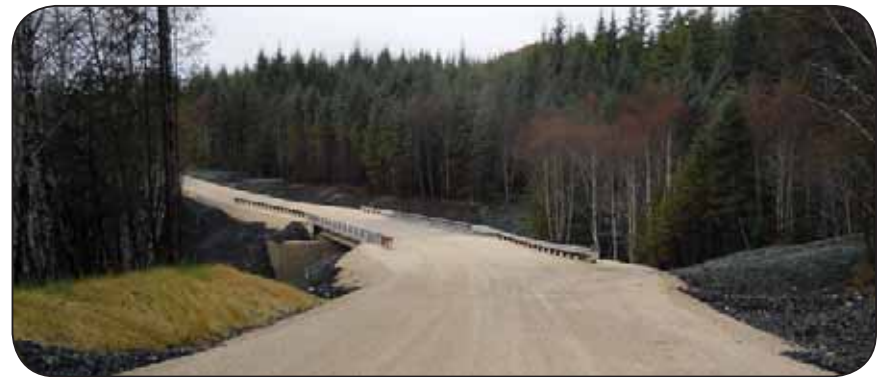
View of approach, Jenny Creek Bridge, Alaska (see FH Project Summary pg 18)
