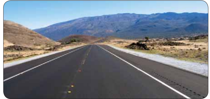
Completed segment, Saddle Road, Hawaii (see Other Title 23 TIGER Project Summary pg 21)
