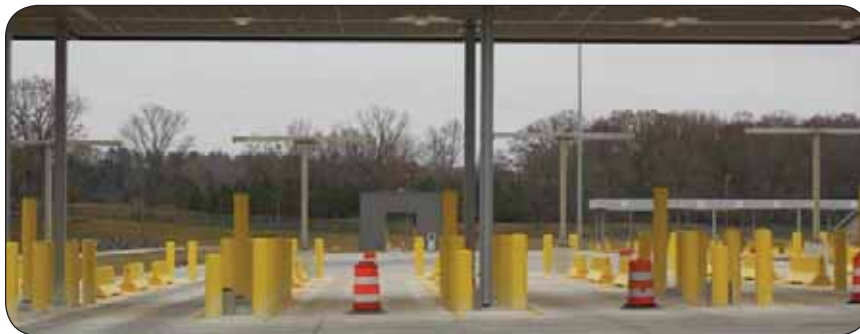
BRIMF outbound and inbound gates with outbound camera portal in background
