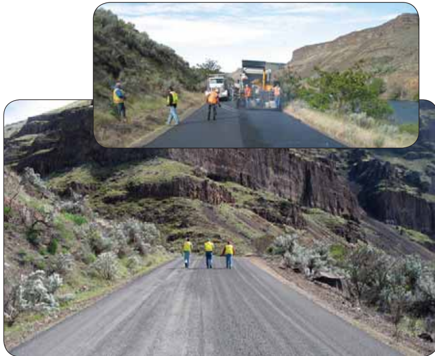
Western Federal Lands review team assessing surface aggregate
