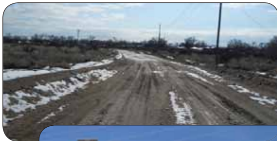
Before — North McCurdy Road, Ohkay Owingeh Pueblo (San Juan Pueblo) Indian Reservation, Espanola, New Mexico. A vital connection for the community, this road was subject to high accident rates and desperately in need of maintenance and safety improvements.
