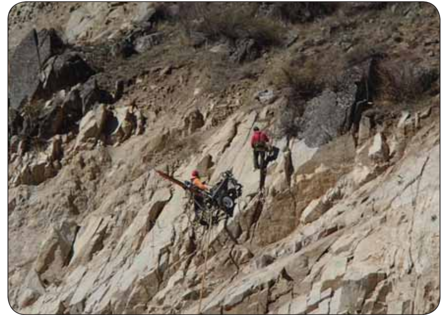
Rock bolt drilling and installation on Banks Lowman Highway, Southwest Idaho, Boise National Forest, an area of frequent, hazardous rockfall in cooperation with Idaho Transportation Department, and Boise County.
