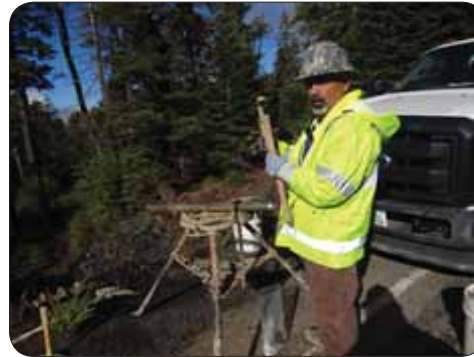
ERFO work, Walker Plains, Plumas National Forest, California
