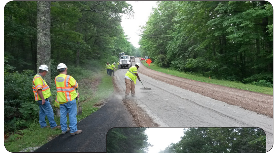
FDR application being observed by VDOT personnel
