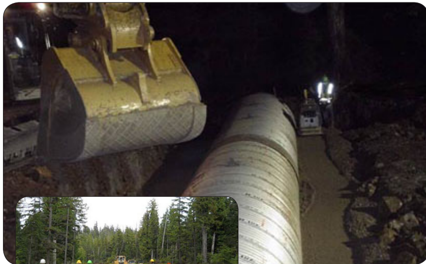
Overnight install of fish pipes
