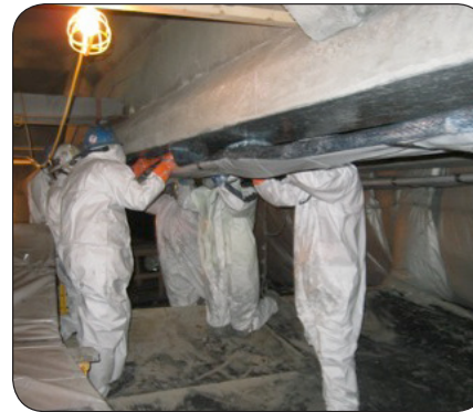
Carbon Fiber Wrap being installed after repair of beam surface
