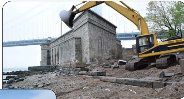
Resetting historic stones
