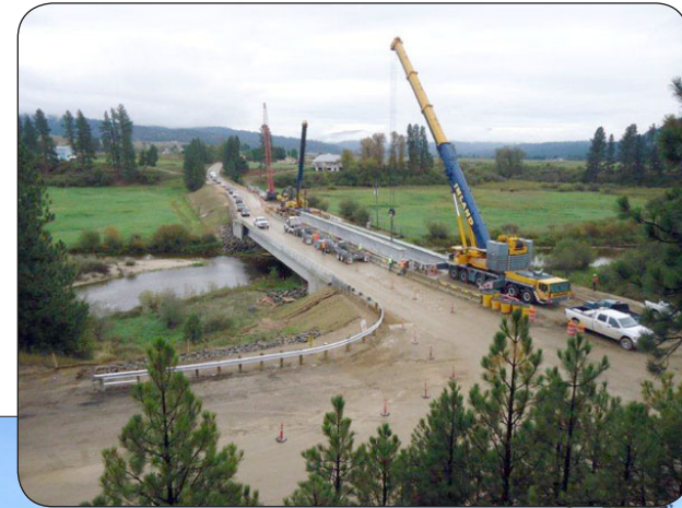
Setting the girders in place
