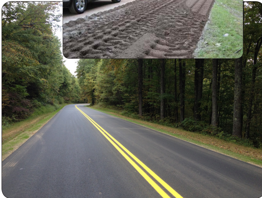
FDR on this project was performed at an 8 inch depth. The NPS was pleased with the process and the quality of the finished roadway and fully supports use of FDR on their future projects. Completed Roadway, Blue Ridge Parkway, Virginia.
