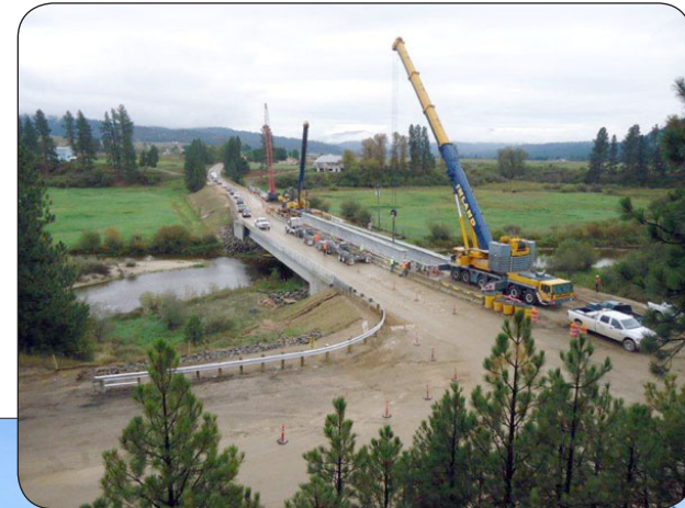
Setting the girders in place
