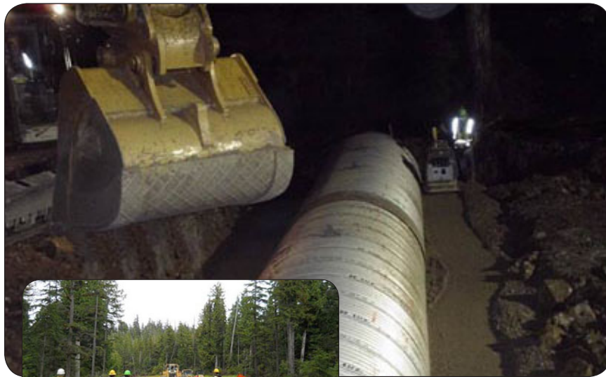
Overnight install of fish pipes
