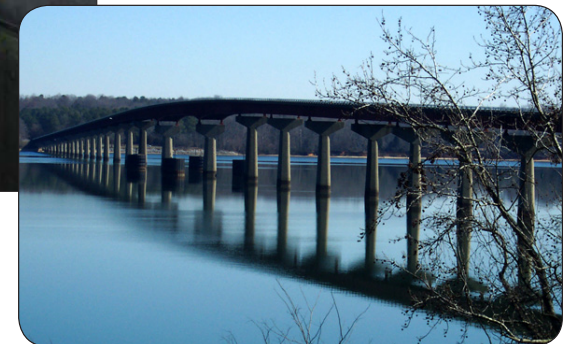
John Coffee Memorial Bridge, Tennessee
