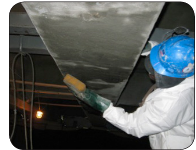
Repair material being applied to bottom of beam
