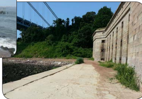
Wall Repaired with Stone Backing
