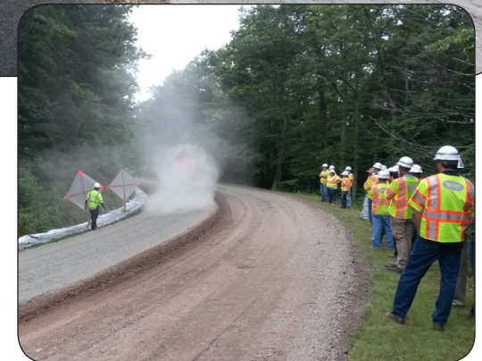
FDR application being observed by VDOT personnel
