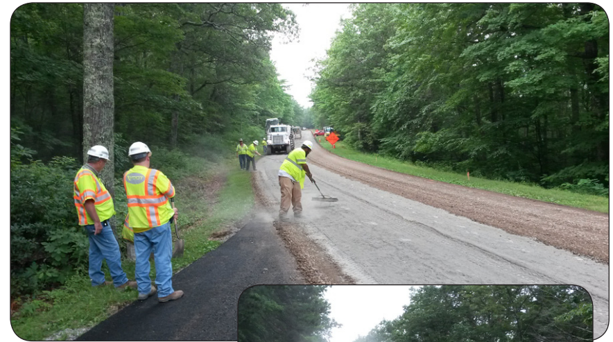
FDR application being observed by VDOT personnel
