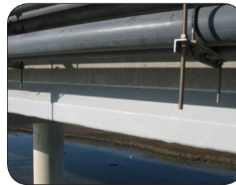
Beam after repaired and finish coat applied
