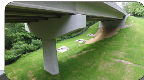
North and South Abutment views show existing rock face and conserved stone used as erosion control.
