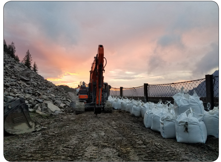
Sand filled “Super Sacks” were used as debris barriers.
