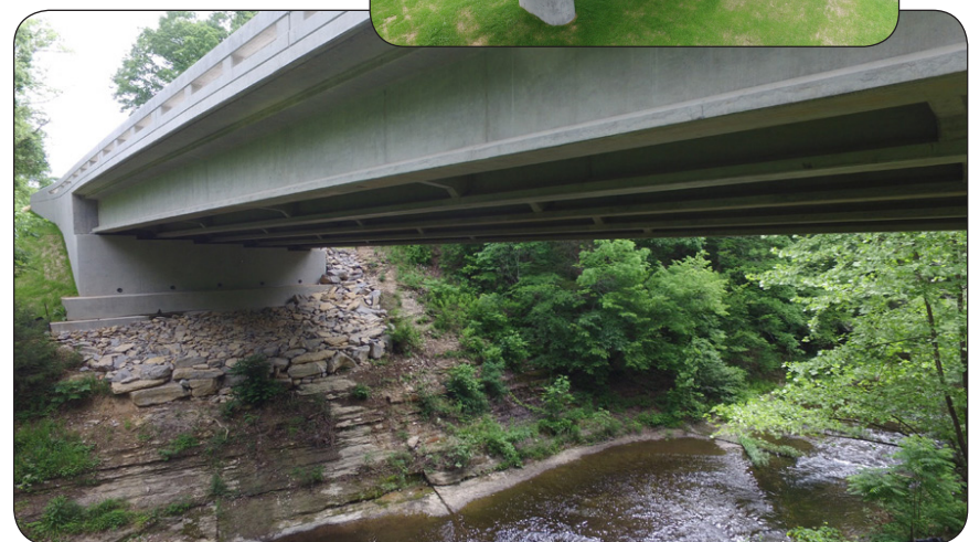
North and South Abutment views show existing rock face and conserved stone used as erosion control.
