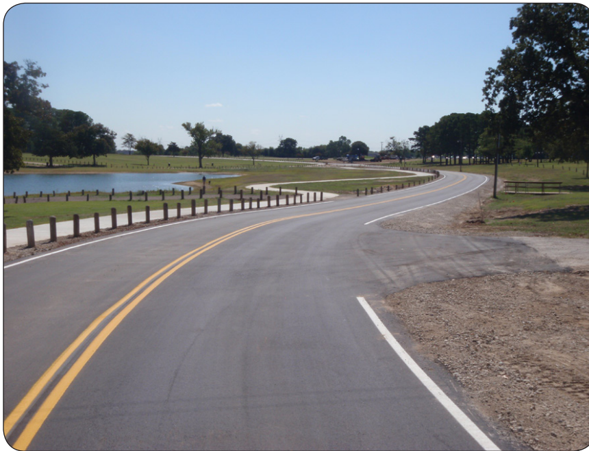
Lake Park Access Road, Lewisville, Texas
