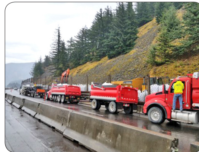
A total of 8,000 feet (4,000 feet for each lane) was moved to create a lane shift away from burnt hill sides.
