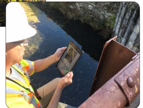
Mobile application in use, C&O Canal National Historical Park, Washington, DC.
