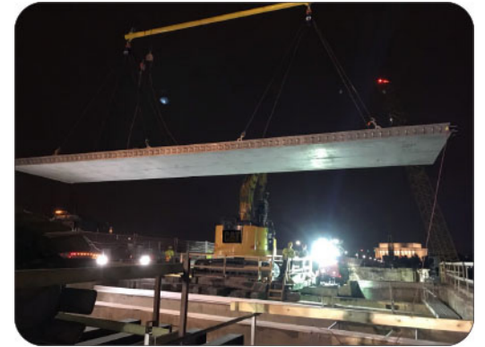
Precast concrete deck installation
