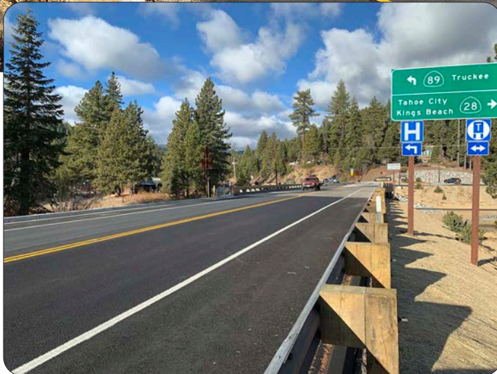
Segment of new section of California State Route 89
