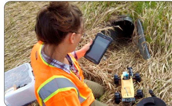
RIP remote controlled tool in use for culvert inspections.
