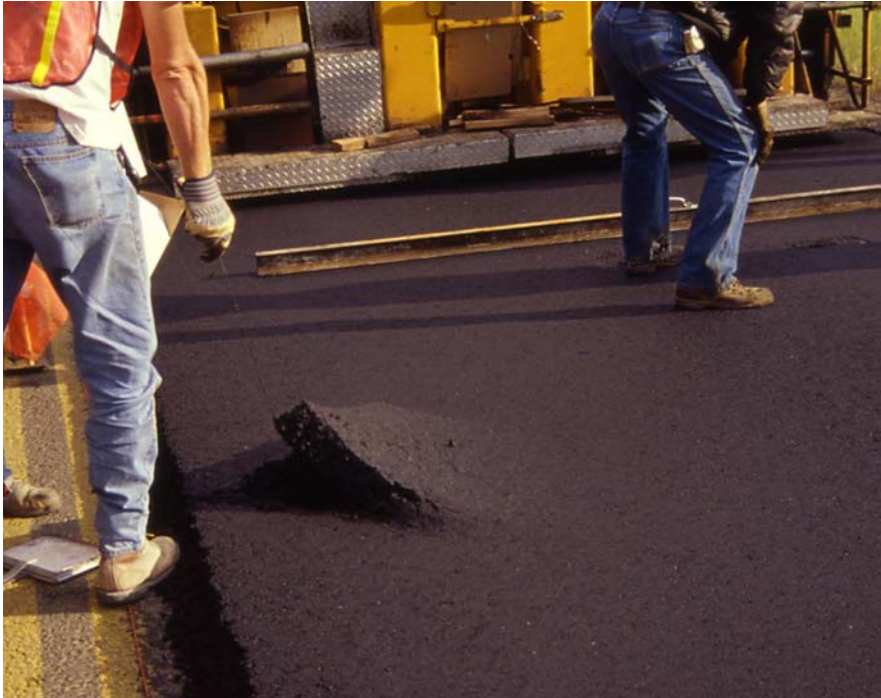
Exhibit 4-5 Obtaining Mixture Sample Prior to Compaction
