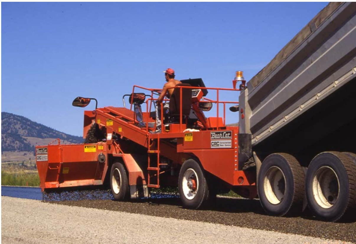
Exhibit 4-12 Chip Seal Aggregate Placement
