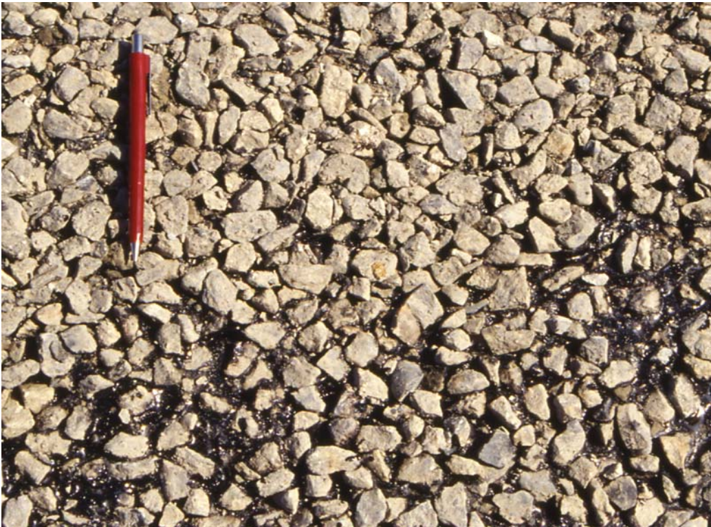
Exhibit 4-14 Completed Chip Seal Surface
