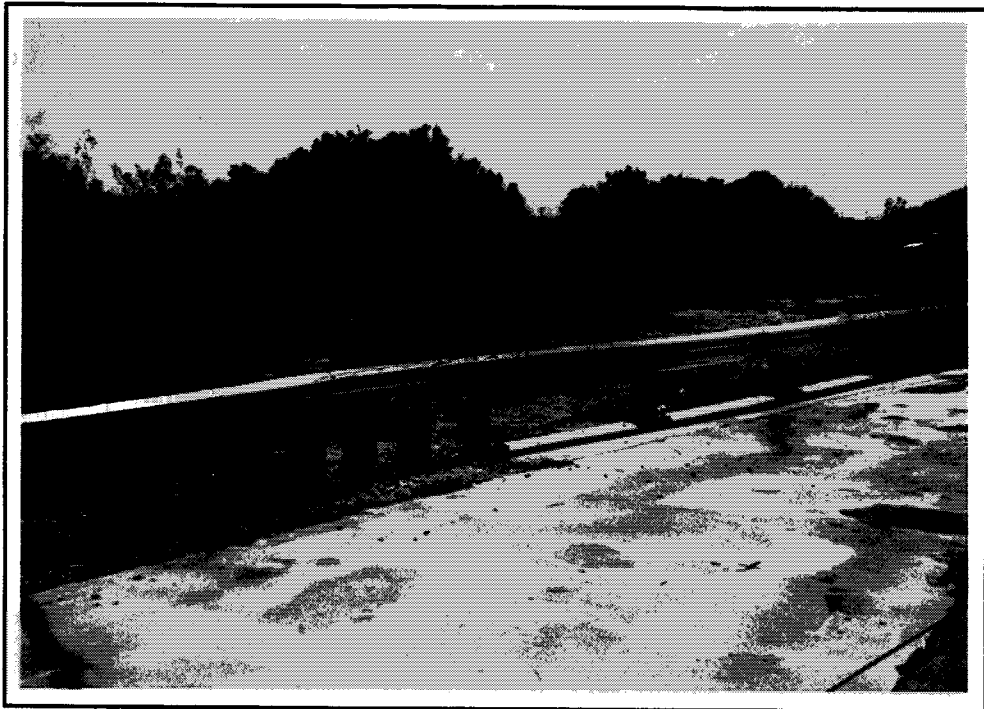
Figure 9. (Continued) After Test Photographs
