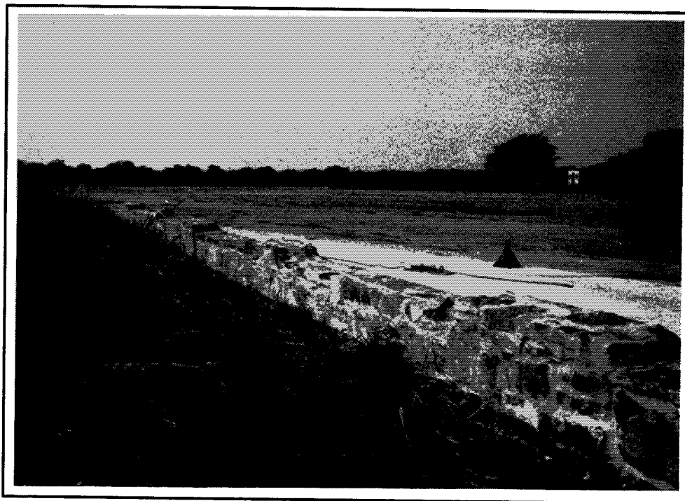
Figure 34. (Continued) After Test Photographs - Test RW-5
