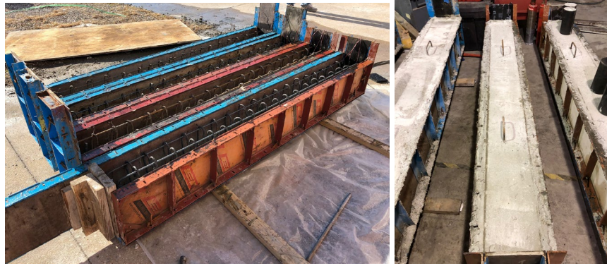
Figure 2-16 – Formwork and cast beams
