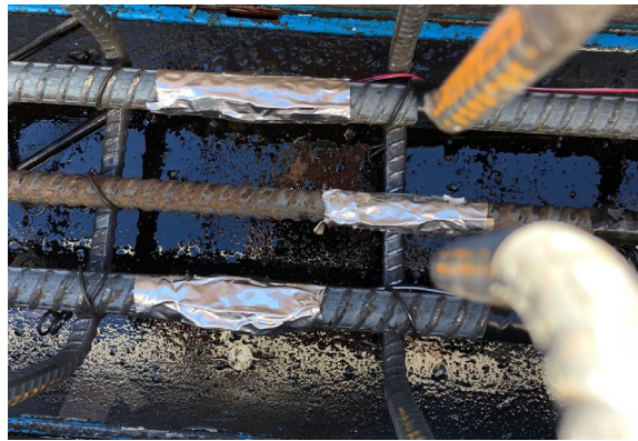
Figure 2-15 – Strain gauges attached at the middle of the bottom reinforcing bars
