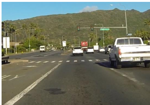
Figure 8-56. Throw-and-roll pothole patch.
