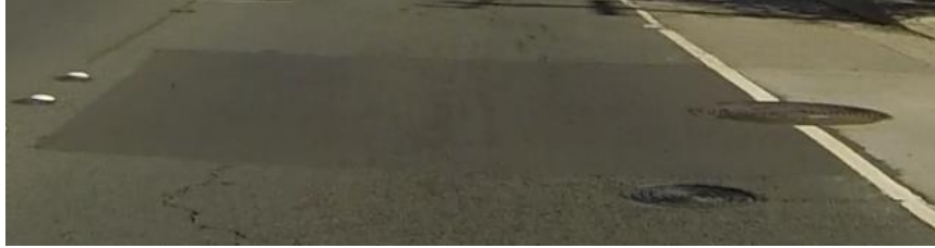
Figure 8-57. Example of a semi-permanent patch.
