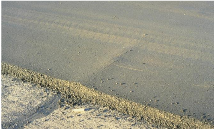
Figure 8-76. Potential problems with sealed cracks
