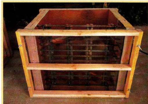
Figure 1: Trial Placement 1 cuyd Form with Reinforcing Cage Matching Drilled Shaft Reinforcement
