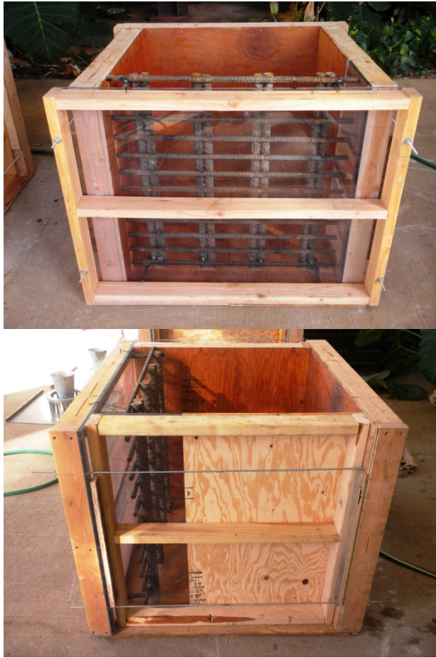
Figure 1: Trial placement 1 cuyd form with reinforcing cage matching drilled shaft reinforcement
