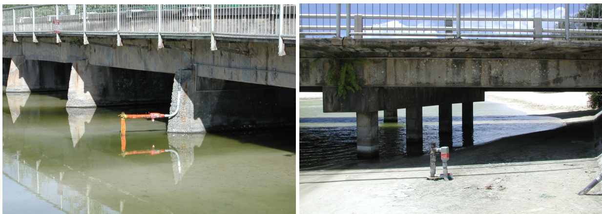
Figure 4-6: The magnetic sliding collars at the middle pier and abutment at Kaelepulu Bridge
