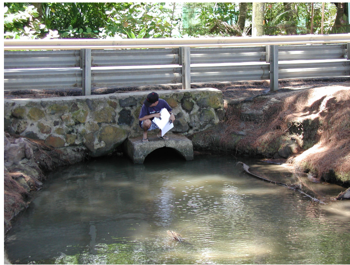
Figure 8-3: Punaluu culvert – 30 in-dia. circular pipe
