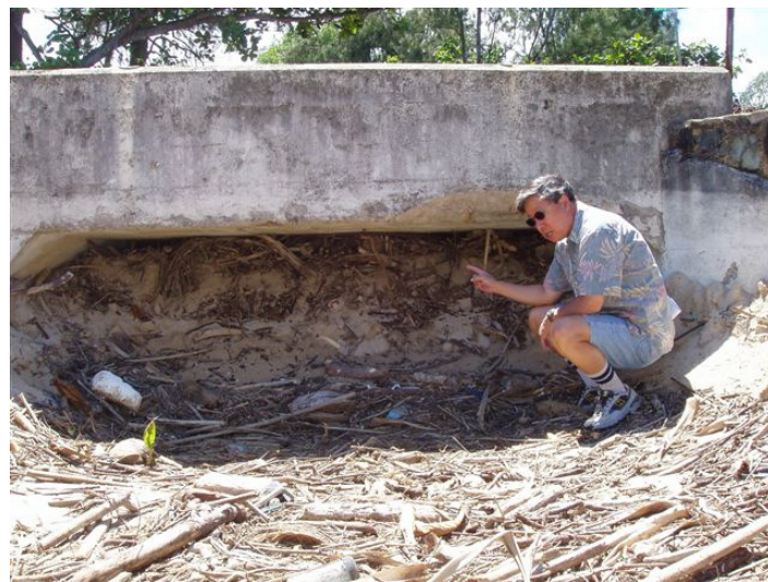
Figure 8-4: Hauula culvert – 6 ft by 8 ft rectangular box
