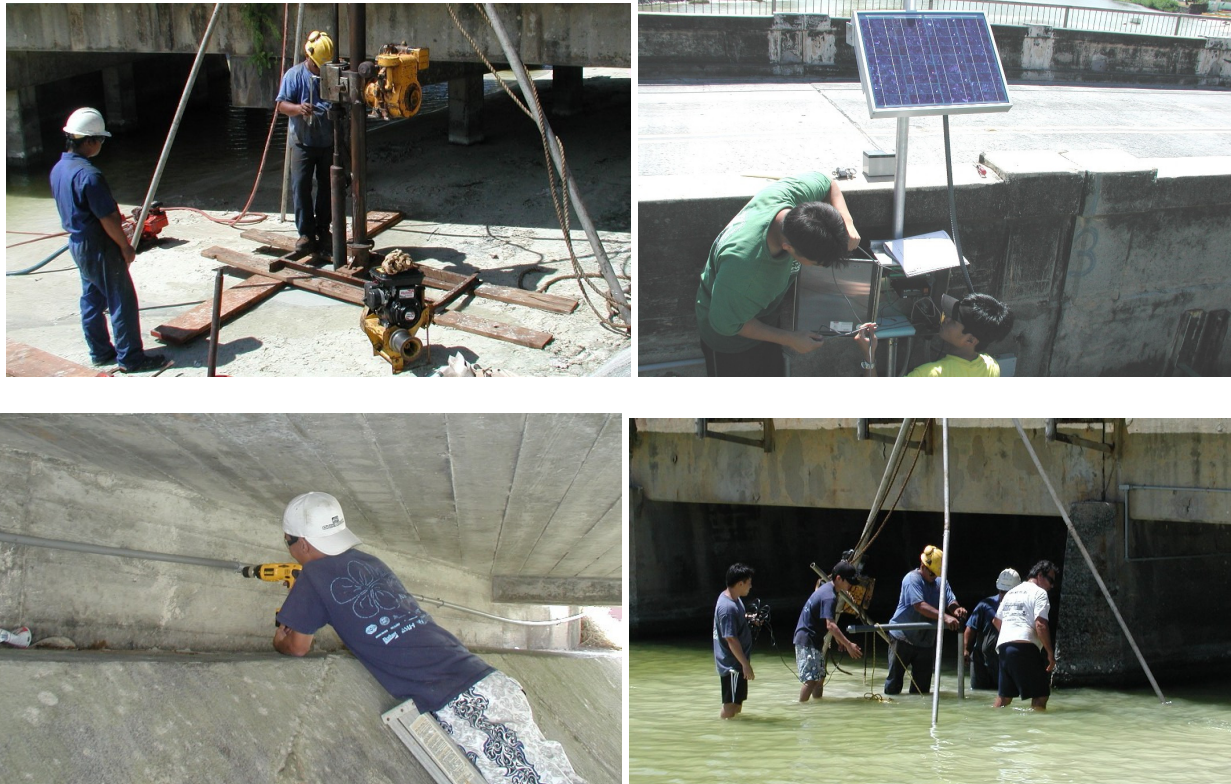
Figure 4-5: Installation of the magnetic sliding collars at Kaelepulu Bridge
