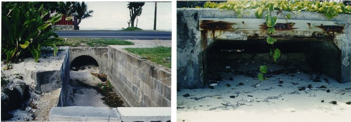
Figure 7-1: Typical sand-plugged culverts on Oahu
