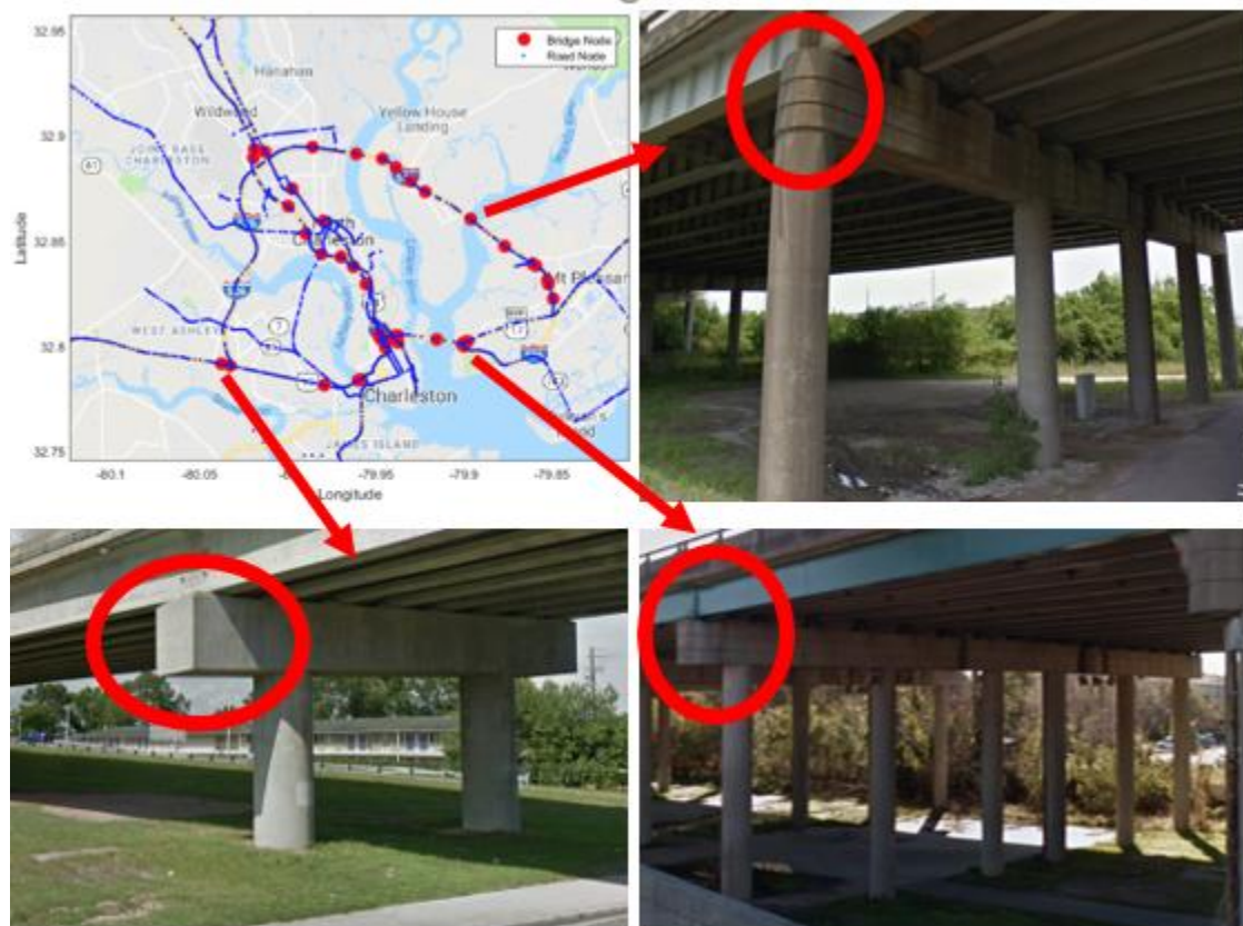
Figure 5.6: Examples of pile-to-bent cap connections
