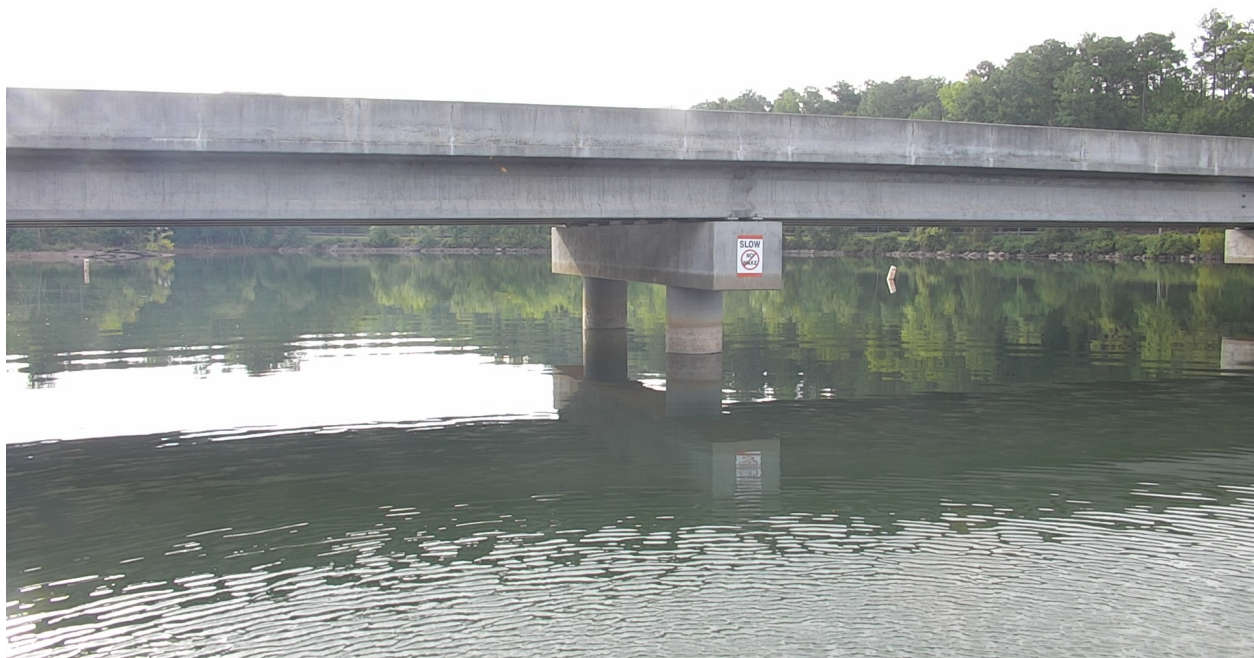
Figure 5.30: Remote test bridge #2.
