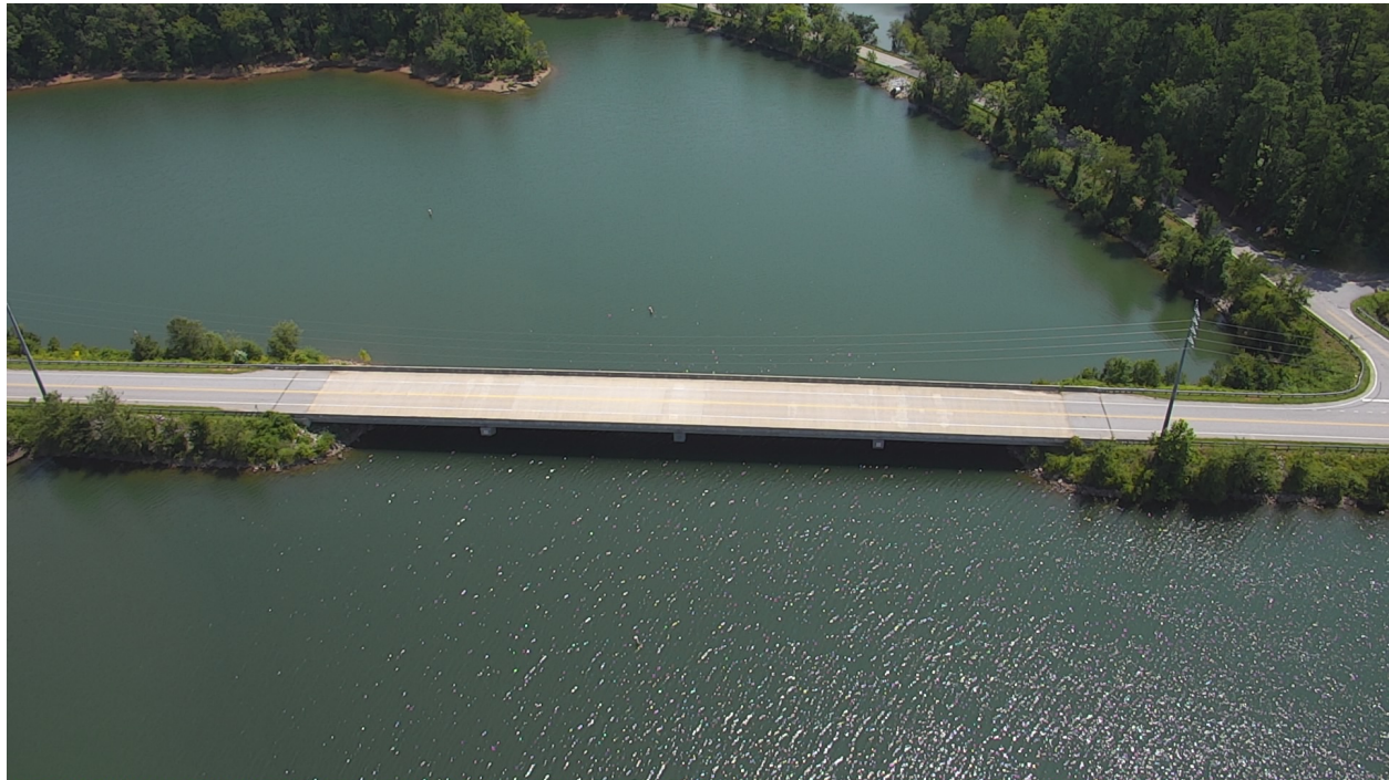
Figure 5.29: Remote test bridge #1.
