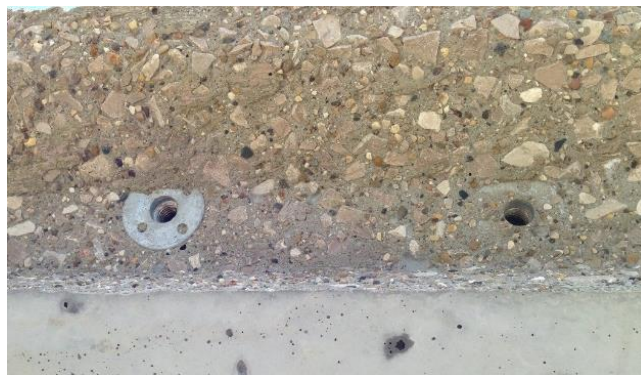
Figure B3: Power Washed Shear Key
