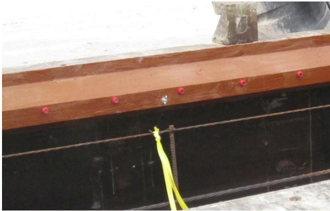
Figure B1: Shear Key Form
