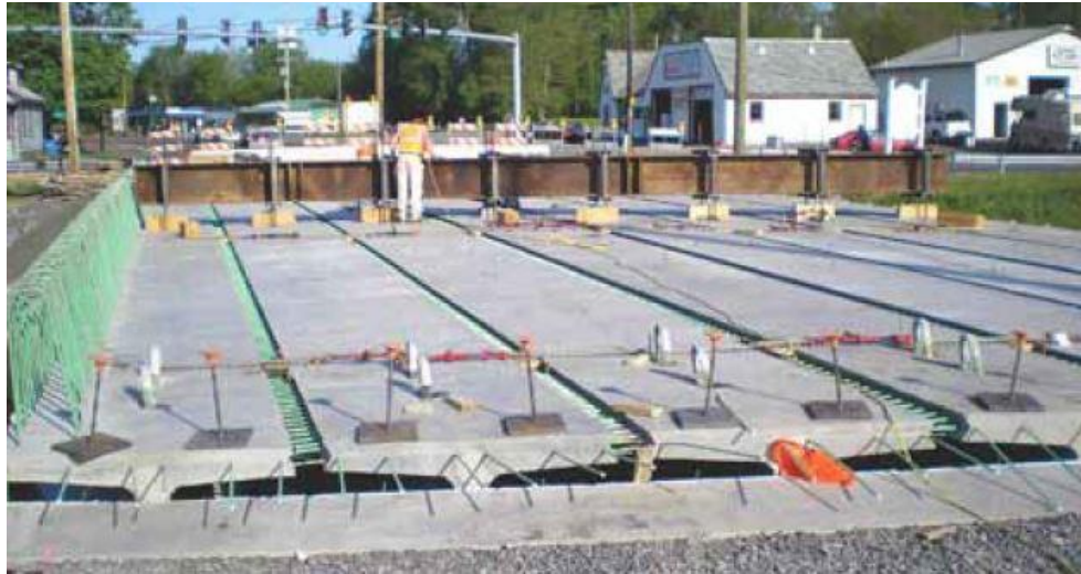
Figure A11: Lyons, NY, DBT Bridge Leveling Operation (Royce, 2011)
