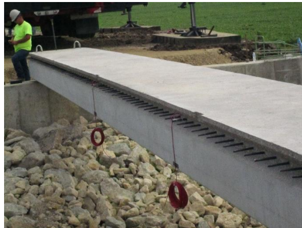
Figure B8: Installed Instrumented Dowel Bars
