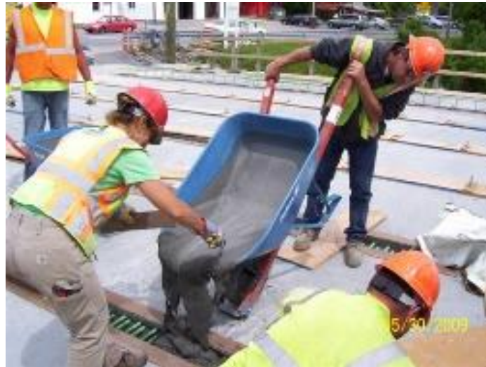
Figure A1: UHPC Placement (Graybeal, 2010a)
