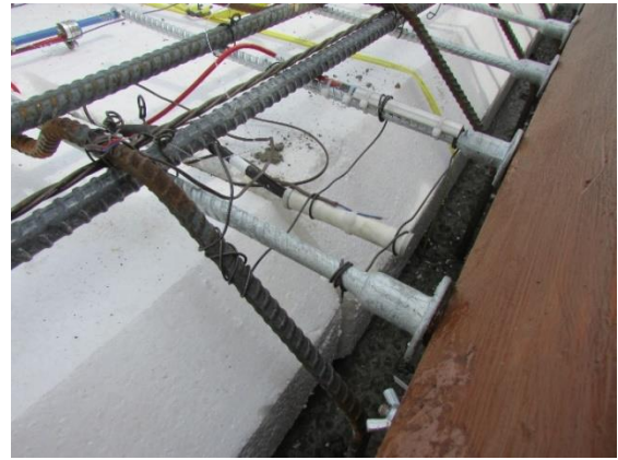
Figure B2: Beam Dowel Parts in Place
