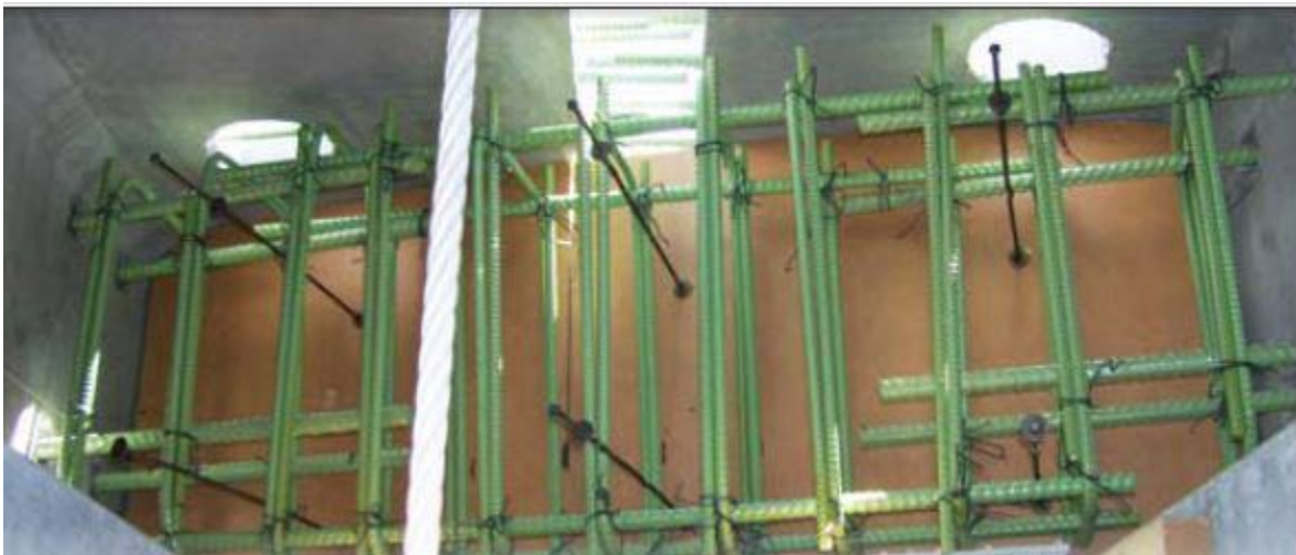
Figure A10: Lyons, NY DBT Bridge from below before UHPC Placement (Shutt, 2009)
