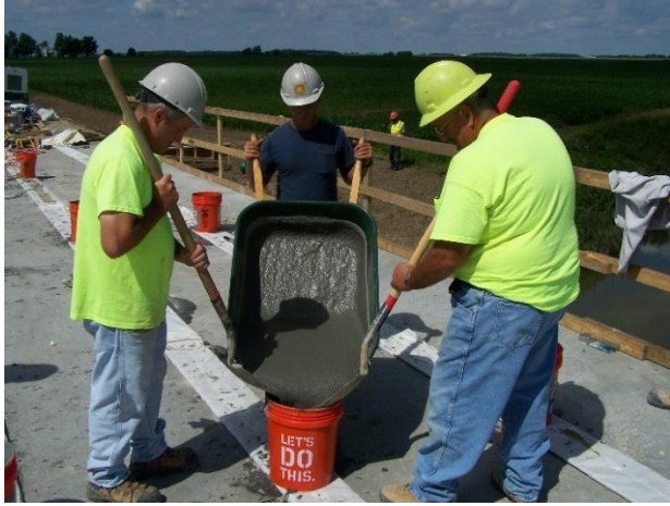
Figure B11: UHPC Placement
