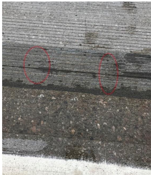
Figure 6: UHPC Cracking
