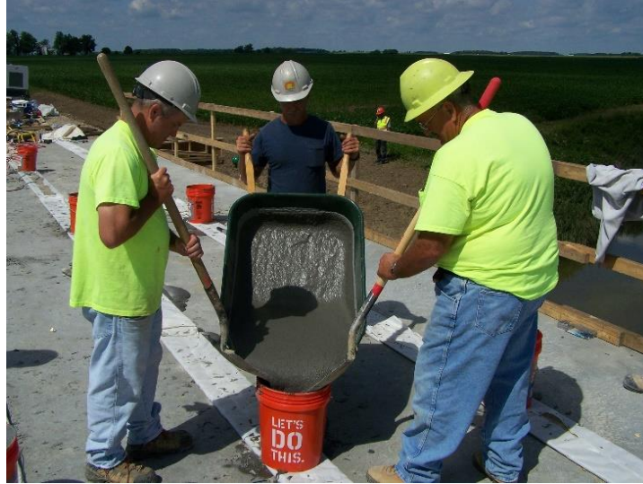
Figure A2: UHPC Placement in Chimneys (Steinberg, et. al., 2015a)
