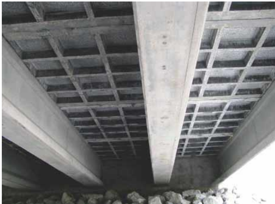
Figure A8: Waffle Deck Panels of Little Cedar Creek Bridge (Moore, 2012)
