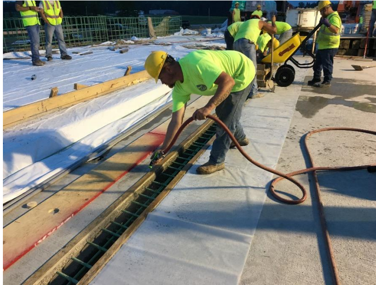
Figure C5: Applying Moisture to Joint
