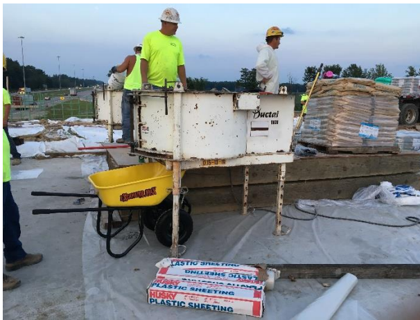
Figure C1: Preparing to Mix UHPC
