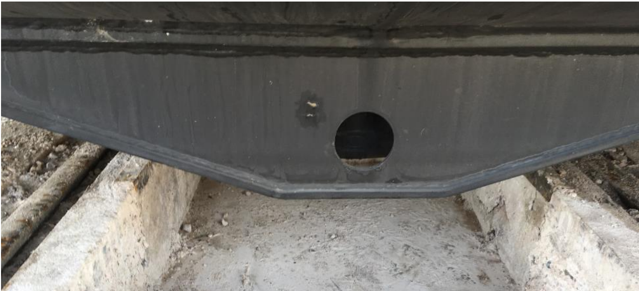
Figure 7. Tank Car's Bottom Valve Protection Structure
